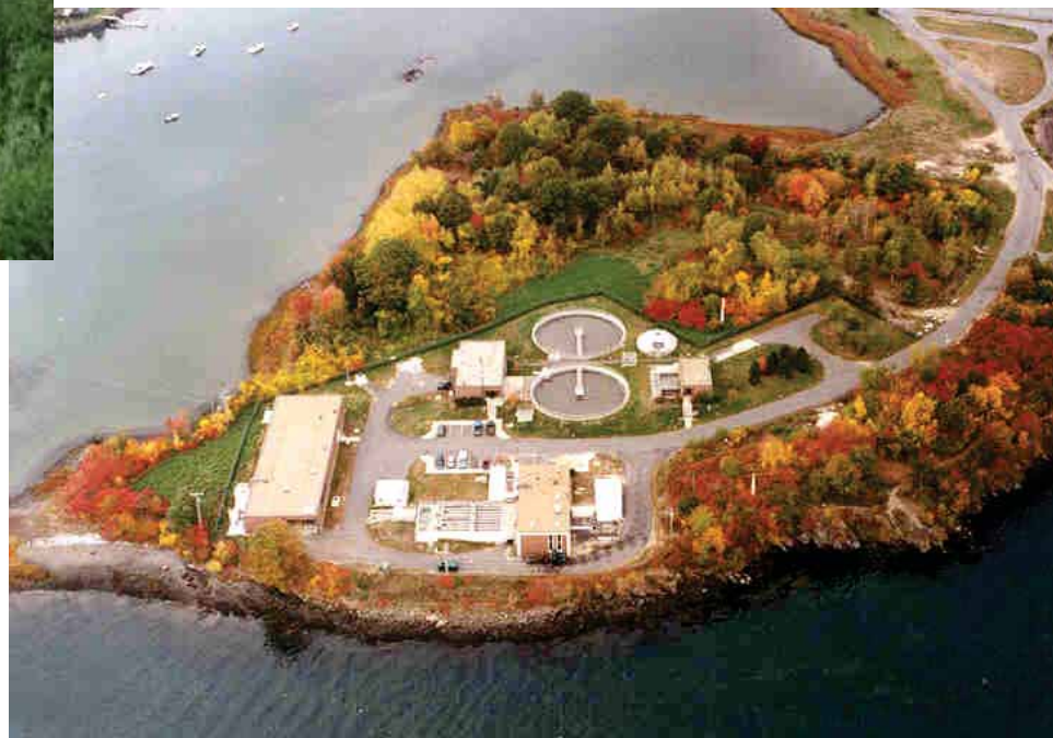
Wastewater Treatment Facilities
