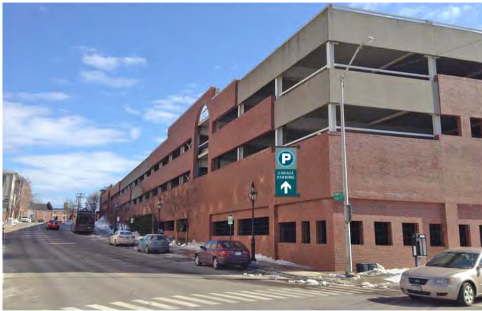
Hanover Garage - Viewing East down Hanover Street
