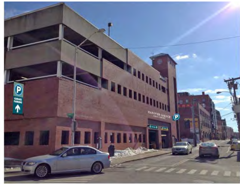
Hanover Garage - Viewing South down Fleet Street
