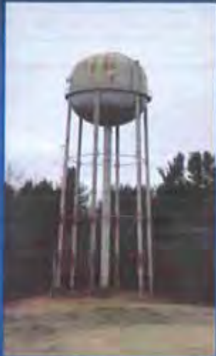
Existing Water Tank
