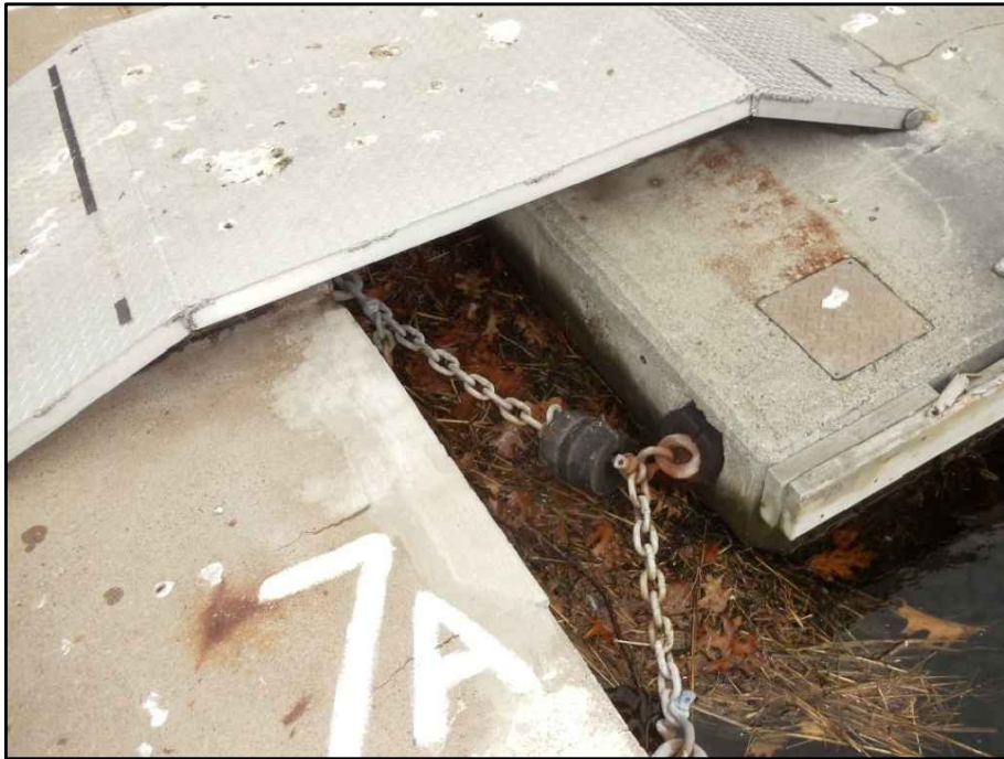
PHOTO 2: FLOATING DOCK CONNECTION
