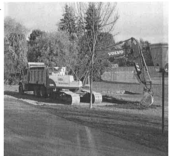
Ground broken for back playground: 10/21/14
