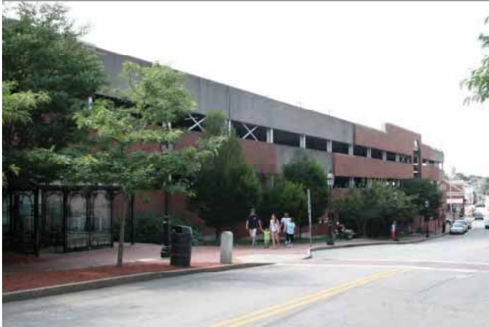
Photo 2 General view – Garage North Elevation
