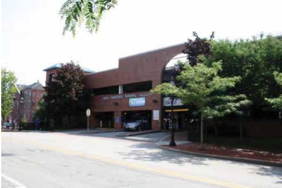
Photo 1 General view – Garage North Elevation
