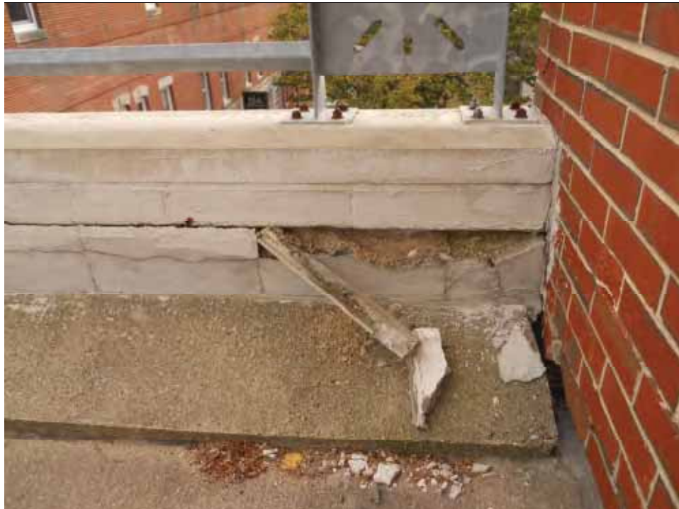
Photo 26 South Elevation. Close view of CMU masonry wall in Photo 25.
