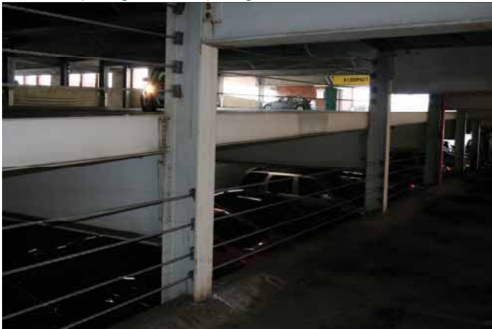
Photo 34 Typical barrier cable guardrailing between floor levels. Note spacing between openings.
