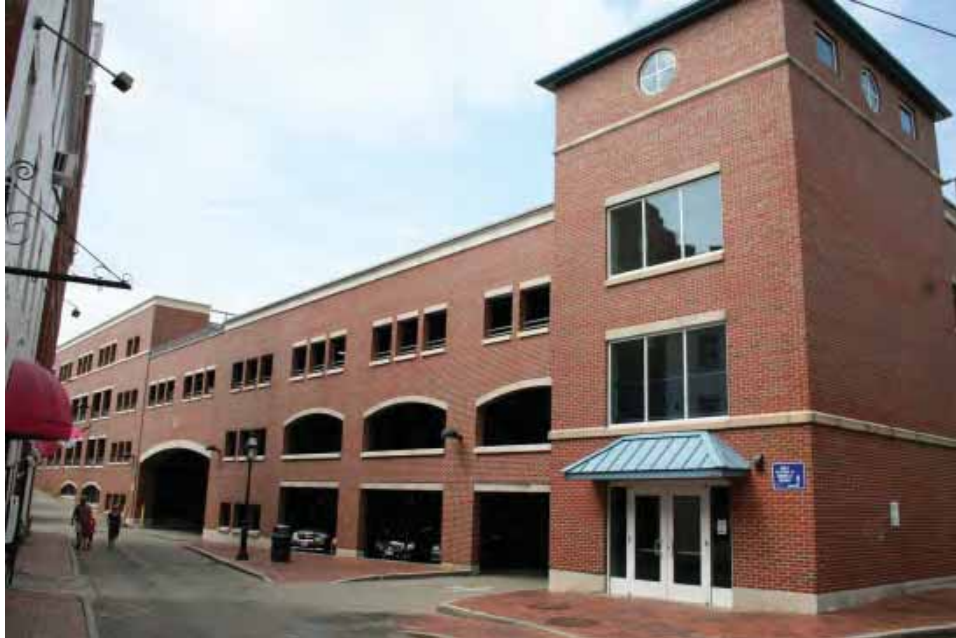
Photo 3 General view – Garage South Elevation
