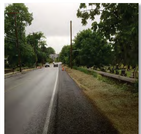
Sagamore Ave. Reconstruction with Porous Pavement
