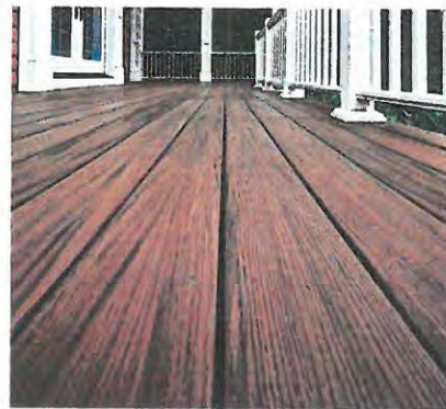
Typical Rear Deck Specification Azek, Arbor Collection Shown Installed with fasteners/plugs ESR-1667
