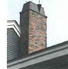
Builder Chimney Face Example 3D No Scale This image displays a faux chimney with brick veneer as built by this builder. Rain pan above will be used, not tall cap.
