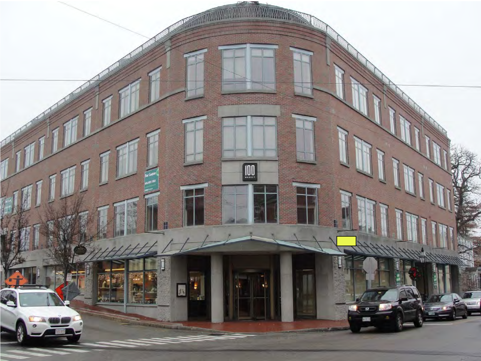
Kahler Chiropractic 100 Market Street 1 Projecting Sign
