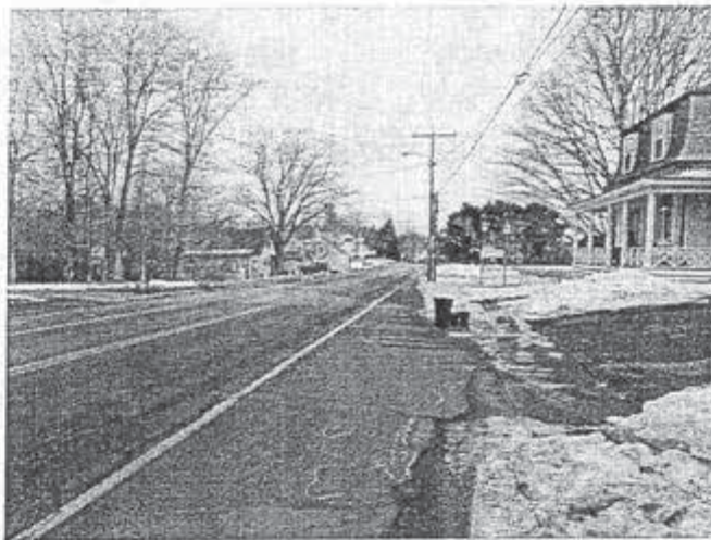
View looking east on Maplewood to downtown over new Maplewood Bridge
