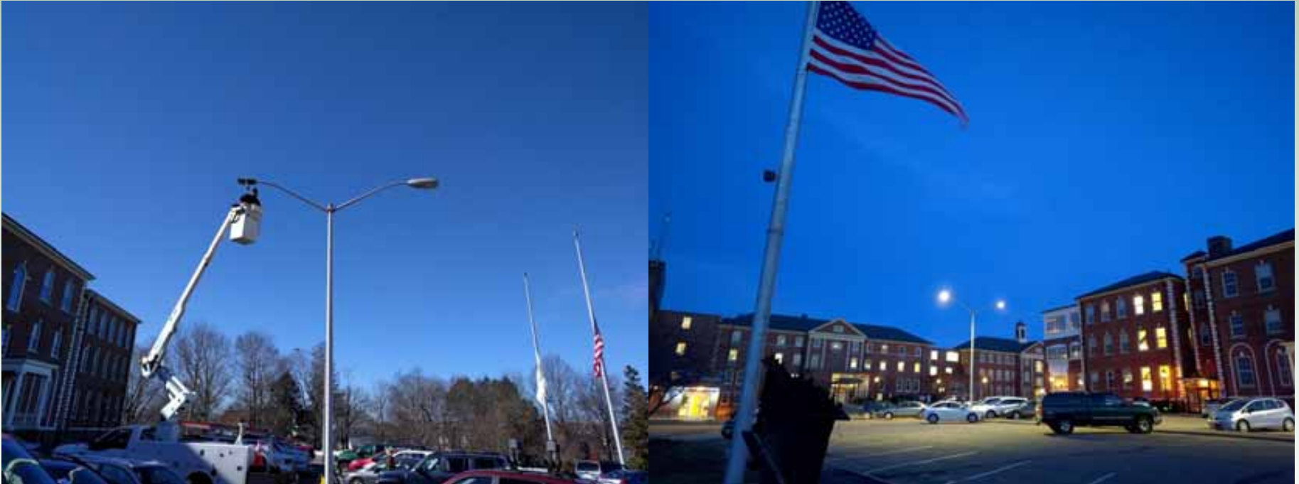
LED Lighting Installation at City Hall
