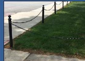
Example Safety Fence Mechanic St and Island
