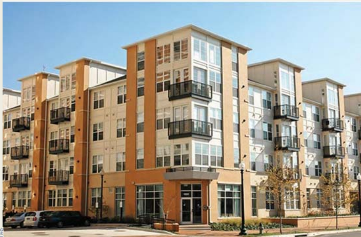
The Silverton in the Silver Spring area of Montgomery County (MD) includes 27 affordable condominiums in a 160-unit complex
