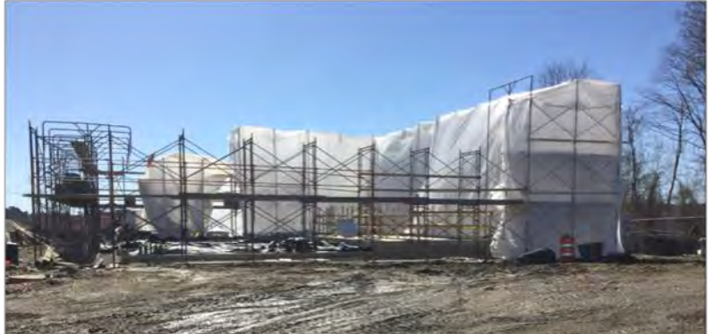
Headworks Building - Under Construction
