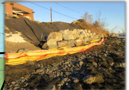
In order to excavate for the new BAF facility, the shoreline had to be stabilized in two locations. This work included installation of large stones to create a stabilized area called a "revetment".
