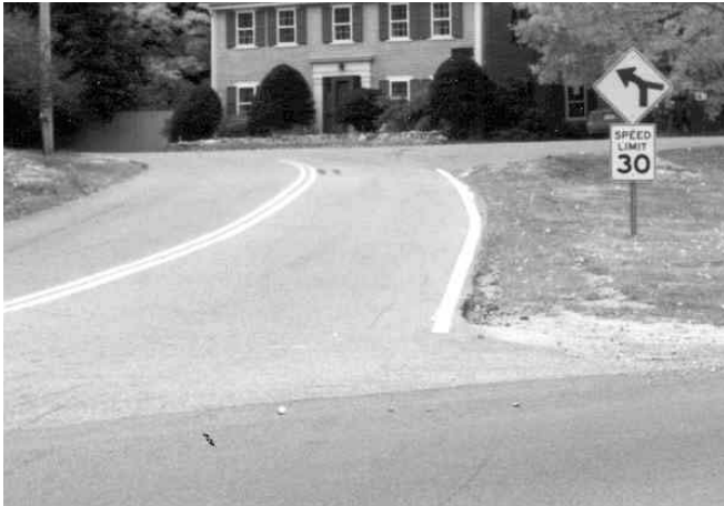
Figure 1. An improperly installed Speed Limit Sign (R2-1)
