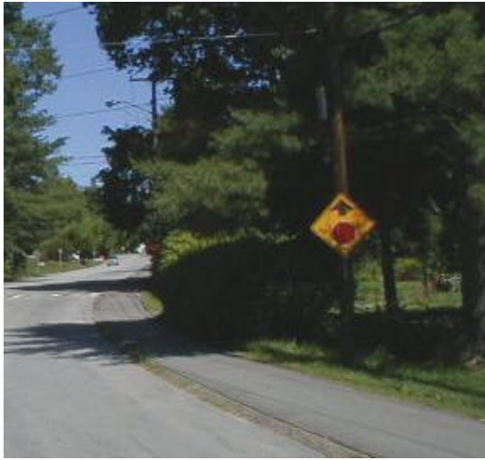
Figure 2. A properly installed Stop Ahead (W3-1a) sign.
