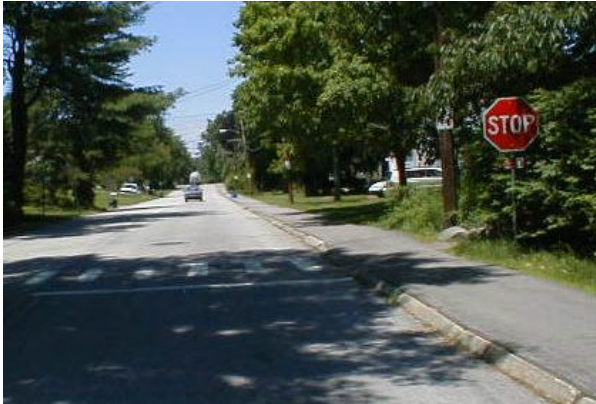
Figure 1. A properly installed STOP(R1-1) sign stop line, and crosswalk.
