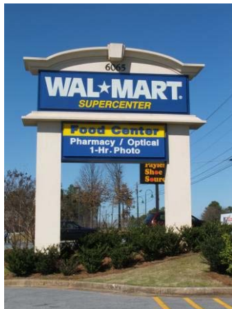
Total width of supports is less than 1/3 of the width of the sign – Not included in sign area
