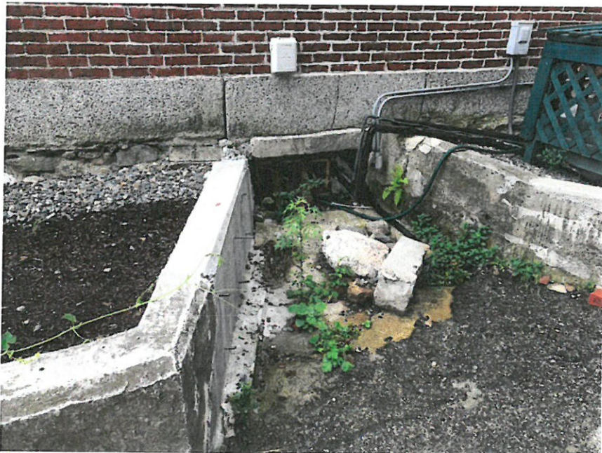
“Bump-In” close-up, showing crack in granite lintel, with jacks supporting.
