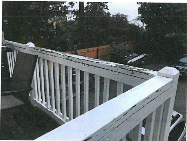
Photo of current painted railing. Railings are composed of 2x4's painted white and square balusters, with accompanying 4x4 posts painted white.
