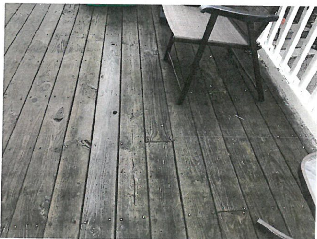
Photo of existing decking. Deck is composed of 5/4x6 pressure treated lumber.
