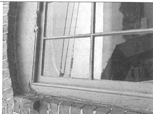
Photo 10: Detail of the window in photo 9. Note the beaded edge.
