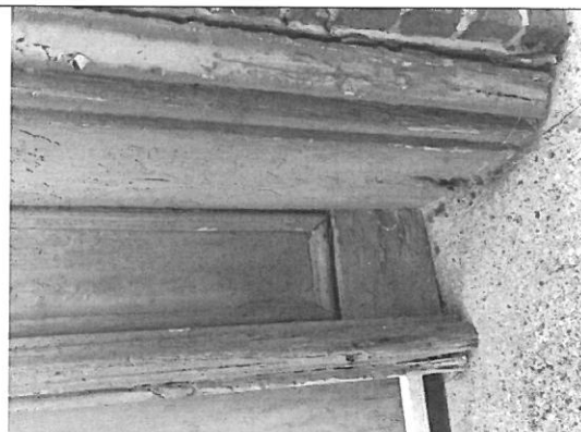
Photo 12: Door A. Detail showing the damaged frame and side panel.
