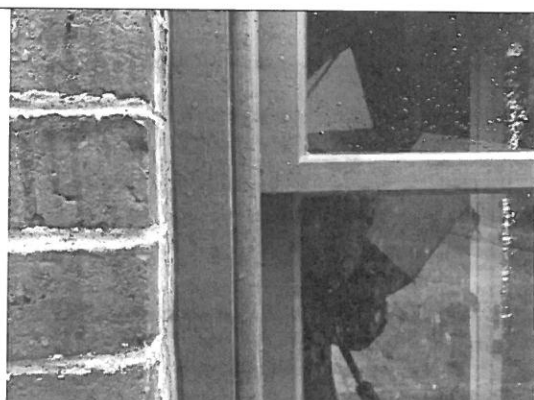
Photo 4: Detail of beaded window frame that replicates historic frames that survive on the building.
