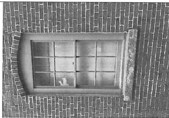
Photo 8: Typical existing window on south elevation. Note the side rails of the frame have been replaced. The majority of the windows have poorly repaired frames like this.
