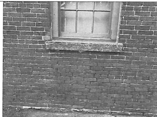
Photo 20: Typical mortar deterioration on the lower four feet of the south facing elevation.
