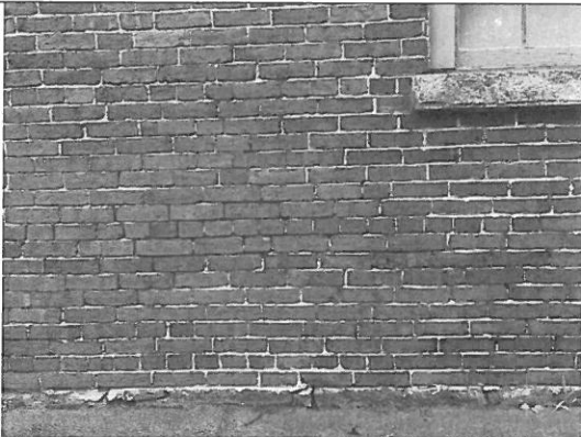
Photo 19: Typical mortar deterioration on the lower four feet of the south facing elevation.
