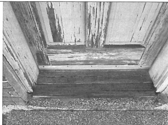
Photo 16: Door C showing the damaged sill.
