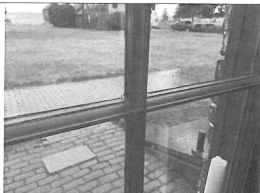
Photo 6: Interior muntin of window installed in 2016.
