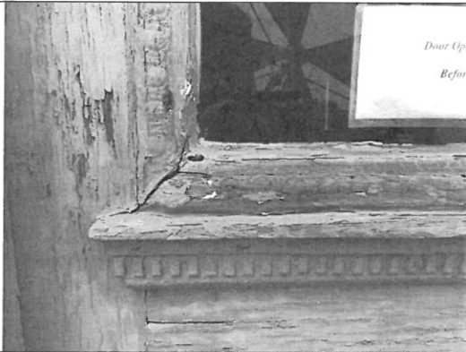
Photo 13: Door A showing damage to the lower frame of the glazed window panel.
