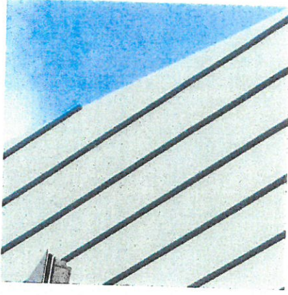
STANDING SEAM METAL ROOF ROOF OF REAR ADDITION
