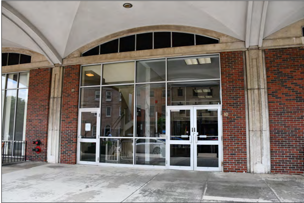
3. South elevation, facing north
