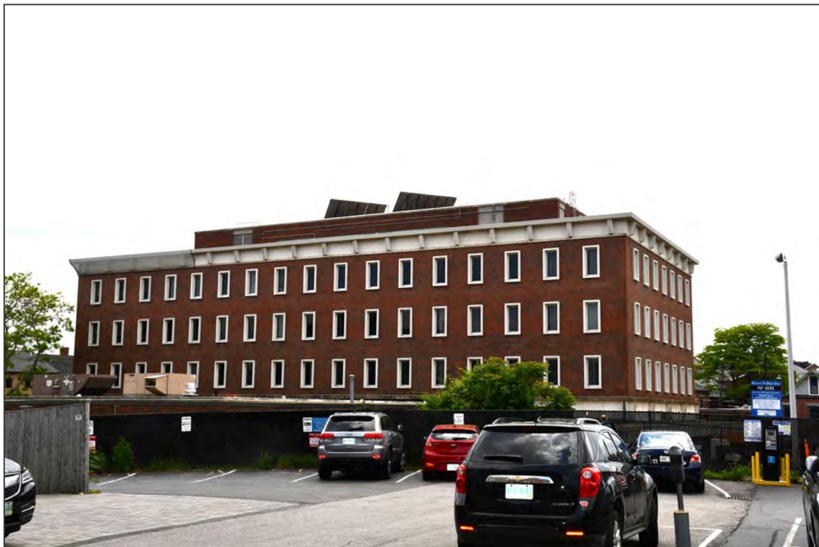
12. East and north elevations, facing southwest
