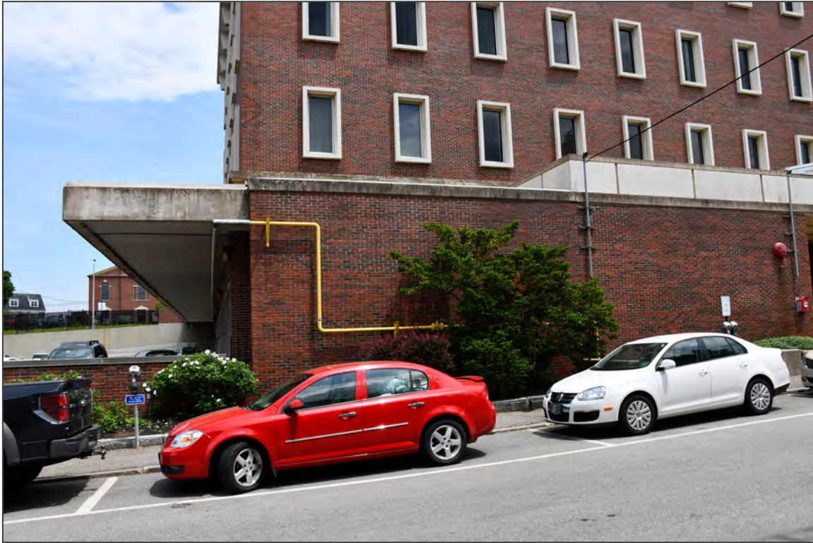
21. West elevation, facing southeast
