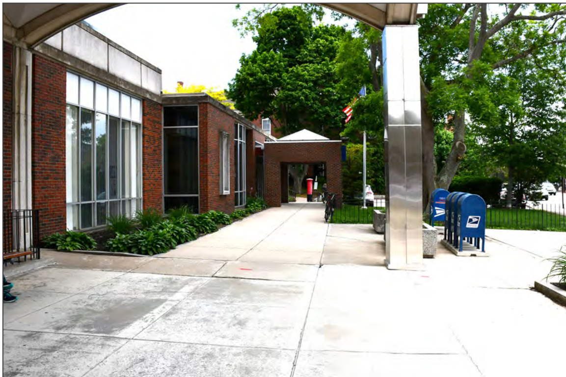
4. South elevation, facing east
