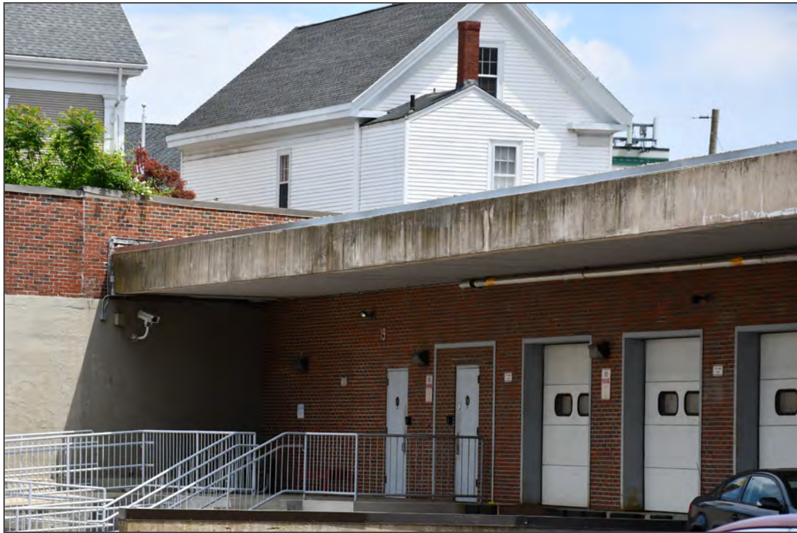
19. North elevation, facing southeast
