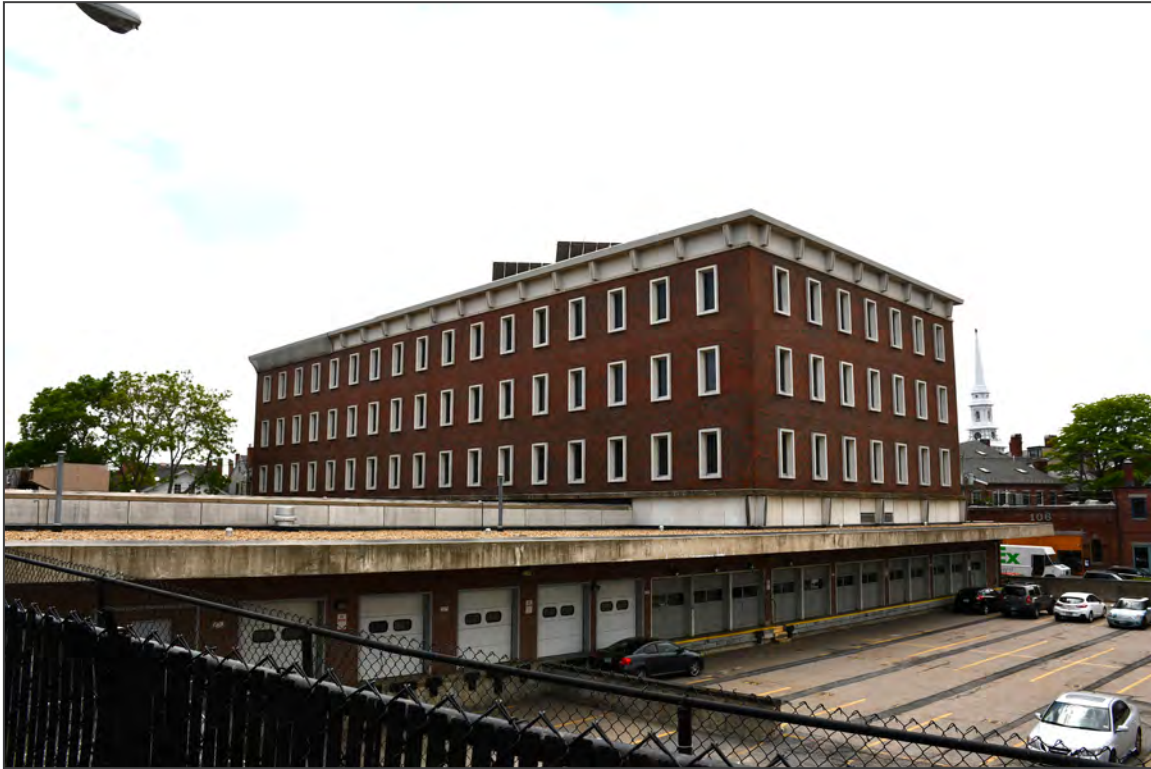
13. East and north elevations, facing southwest
