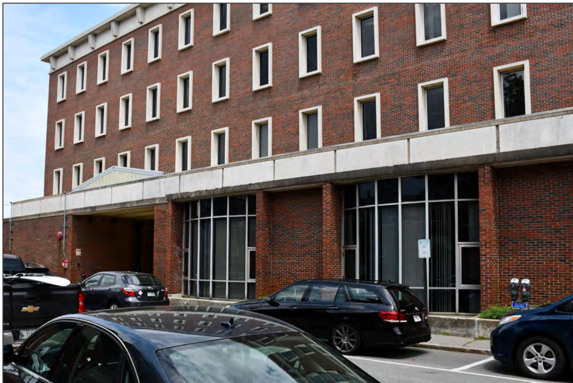
26. West elevation, facing northeast
