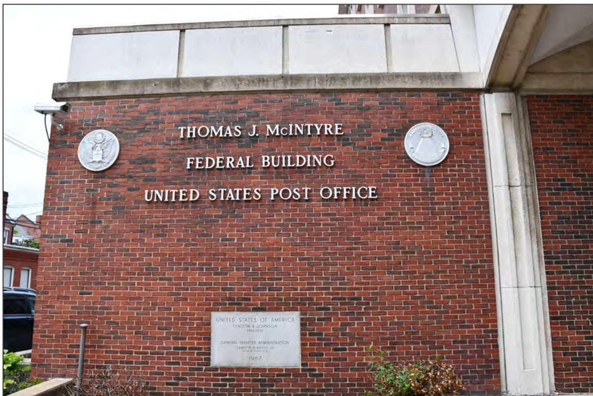
2. South elevation, facing north
