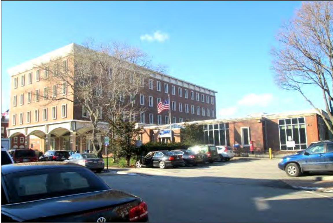
9. South and east elevations, facing northwest
