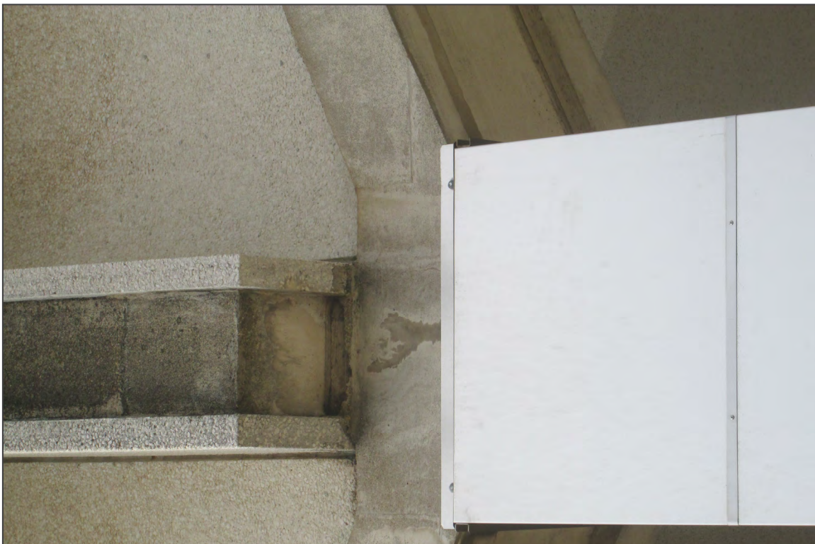
28. South elevation column detail
