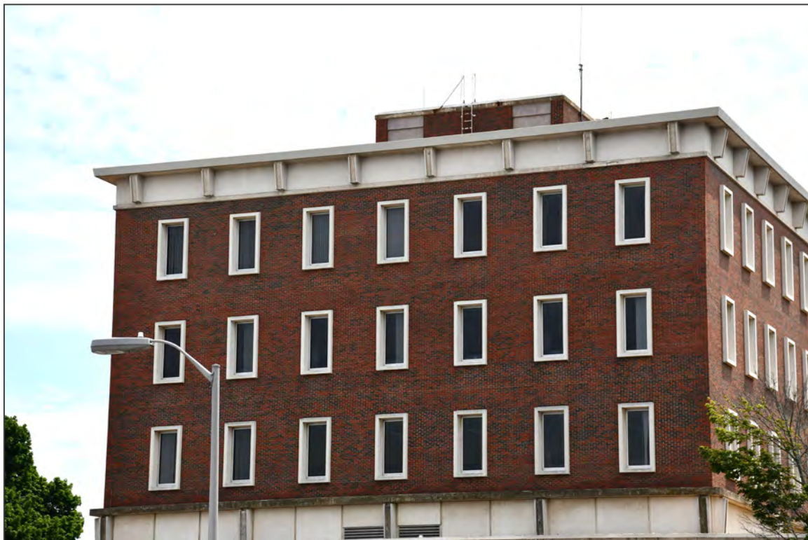
18. North elevation, facing southeast
