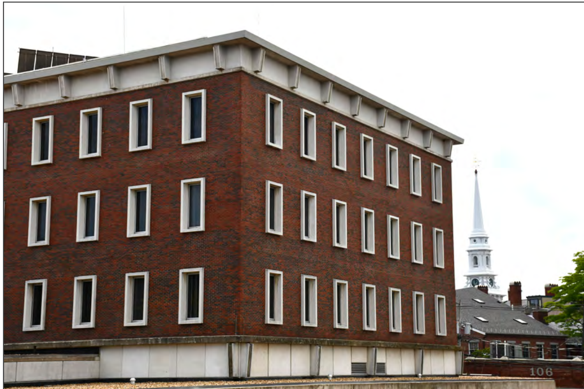
15. East and north elevations, facing southwest
