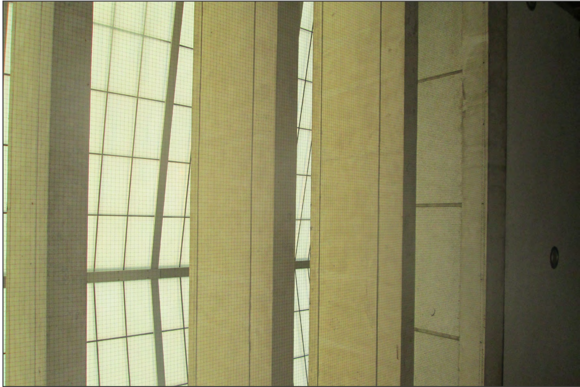
25. West elevation entrance covering
