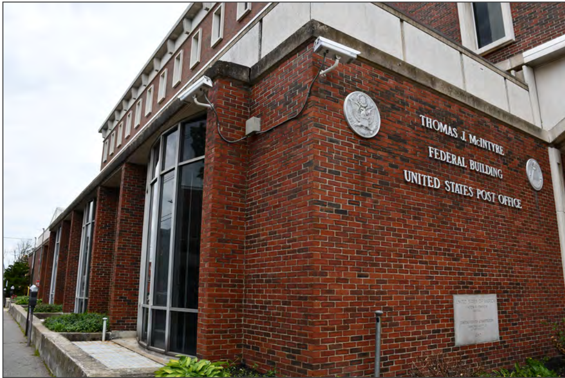
1. West and south elevations, facing northeast
