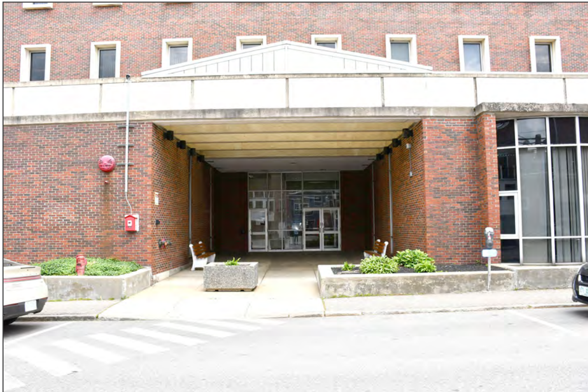
23. West elevation, facing east
