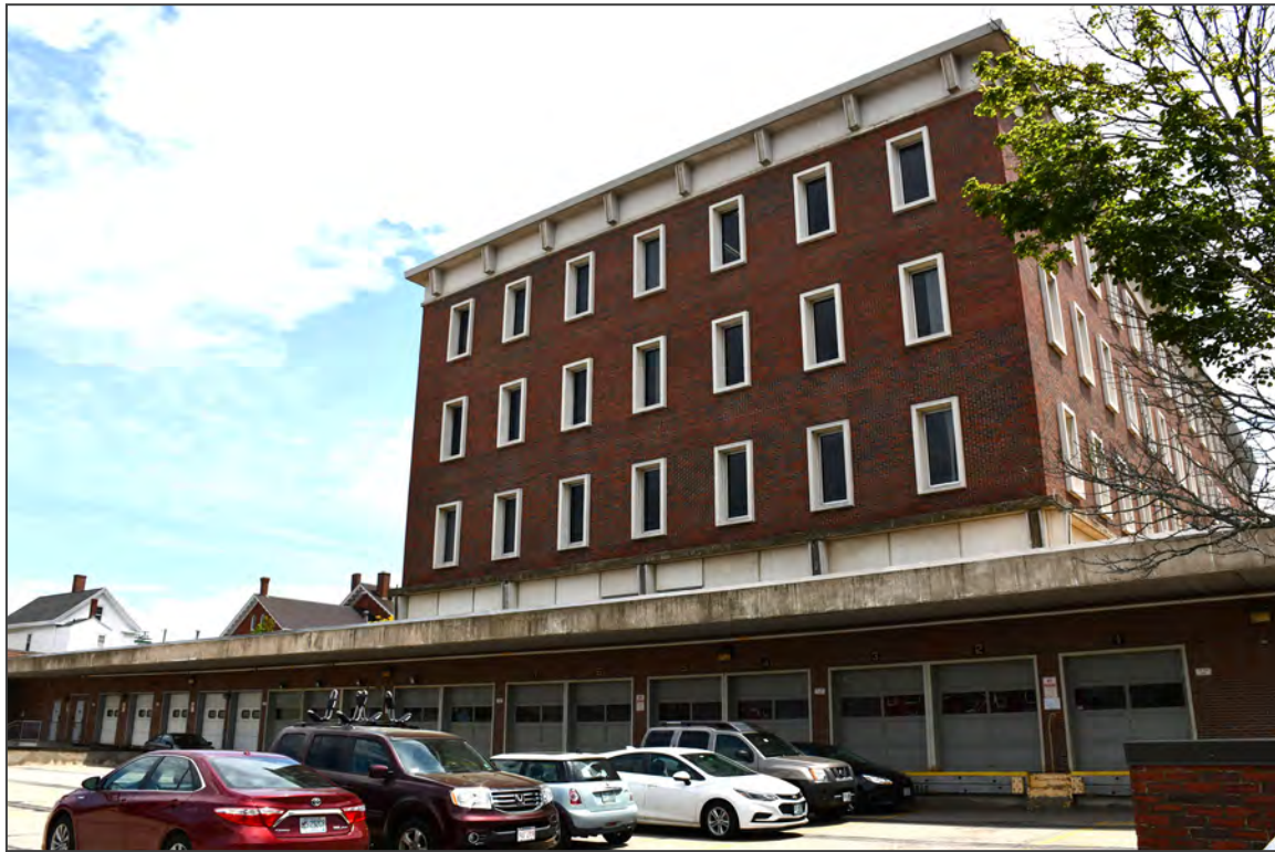
17. North elevation, facing southeast
