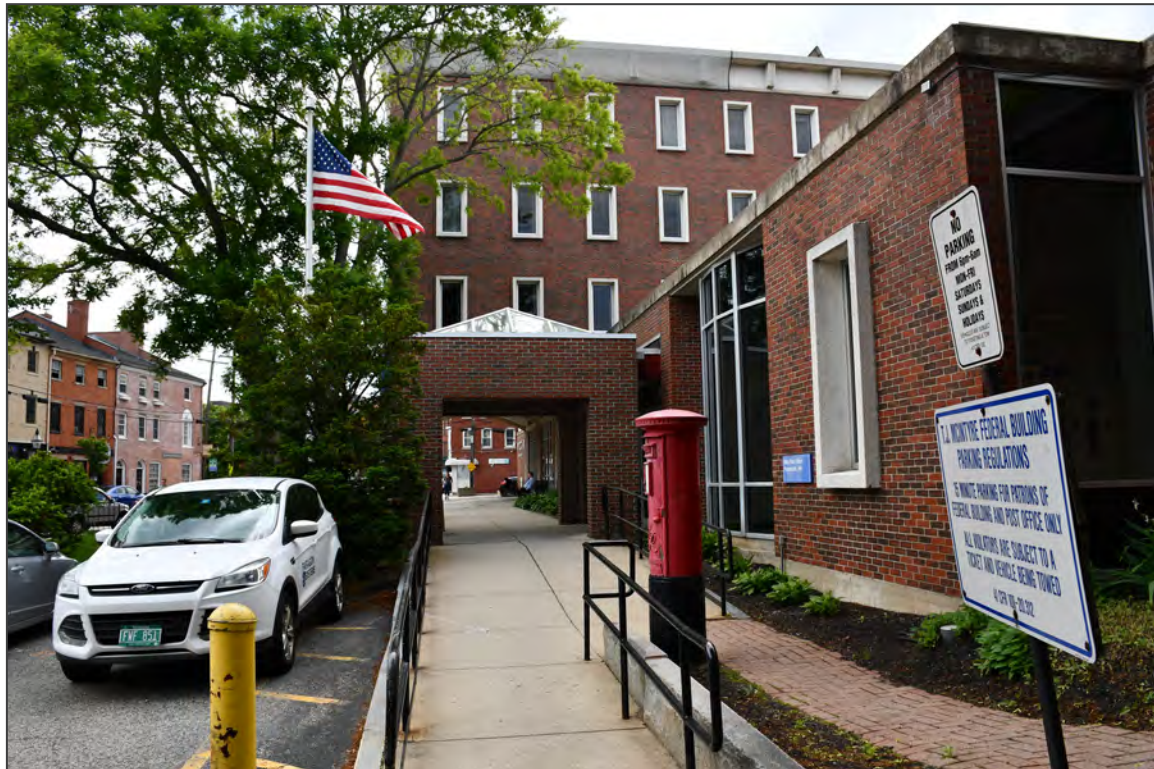
7. East and south elevations, facing west
