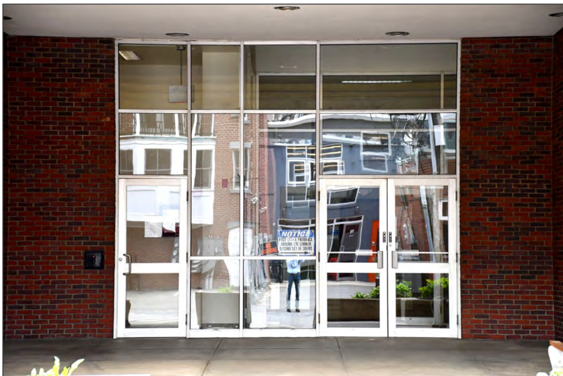
24. West elevation, facing east
