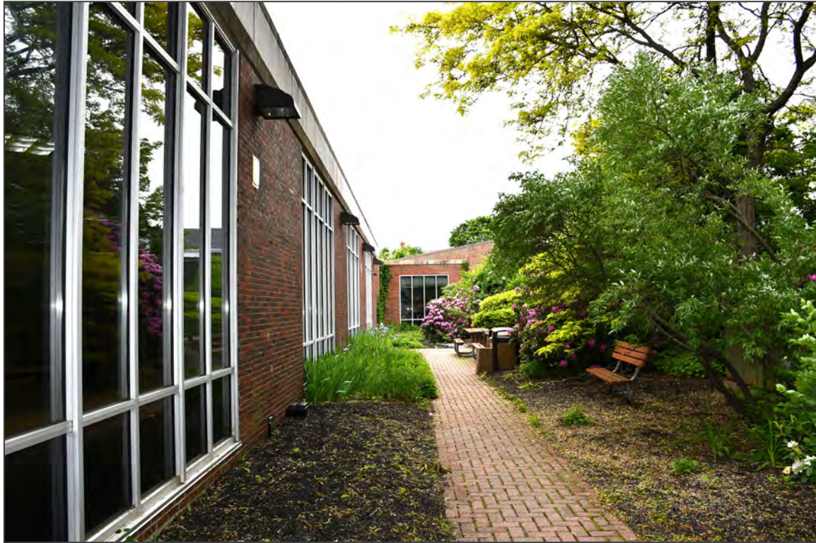
11. East and south elevations, facing north
