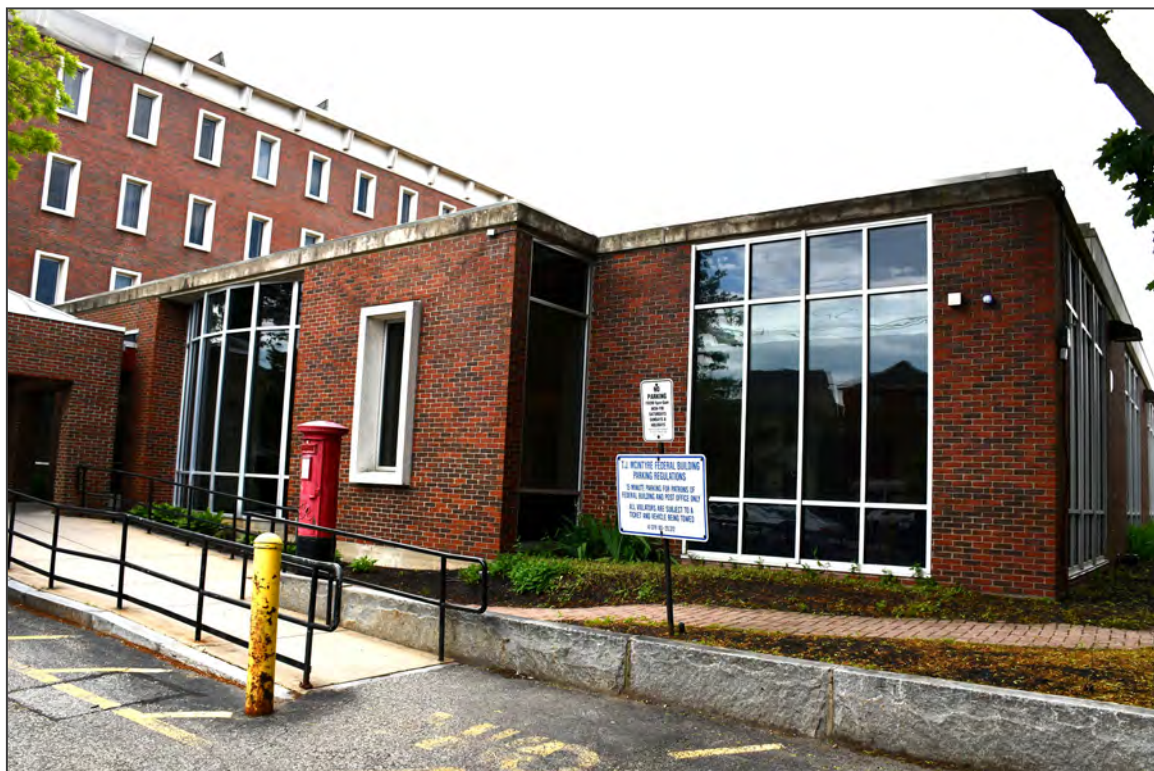
8. East and south elevations, facing northwest
