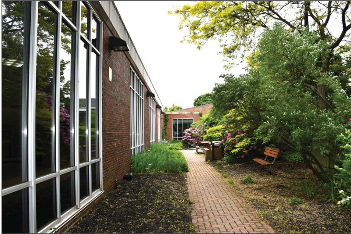
11. East and south elevations, facing north
