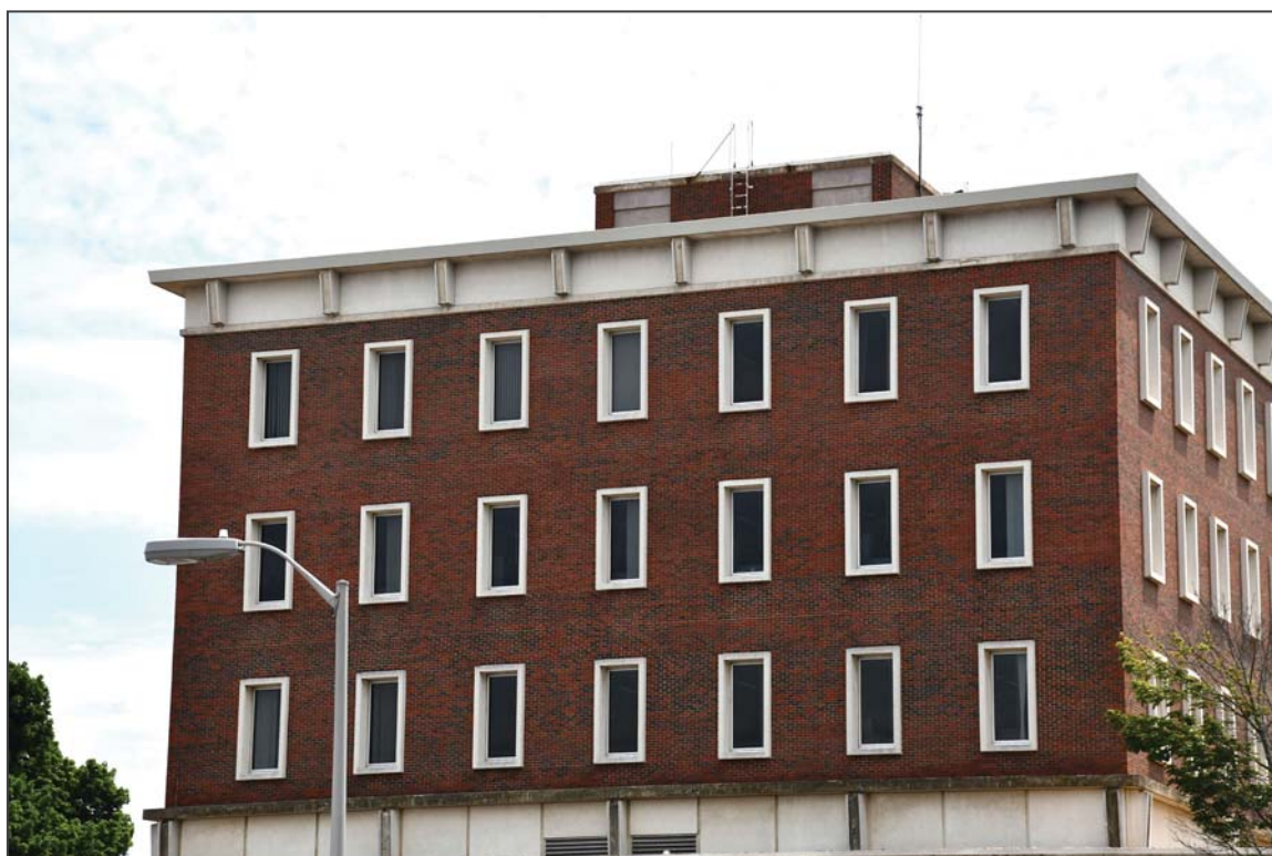
18. North elevation, facing southeast
