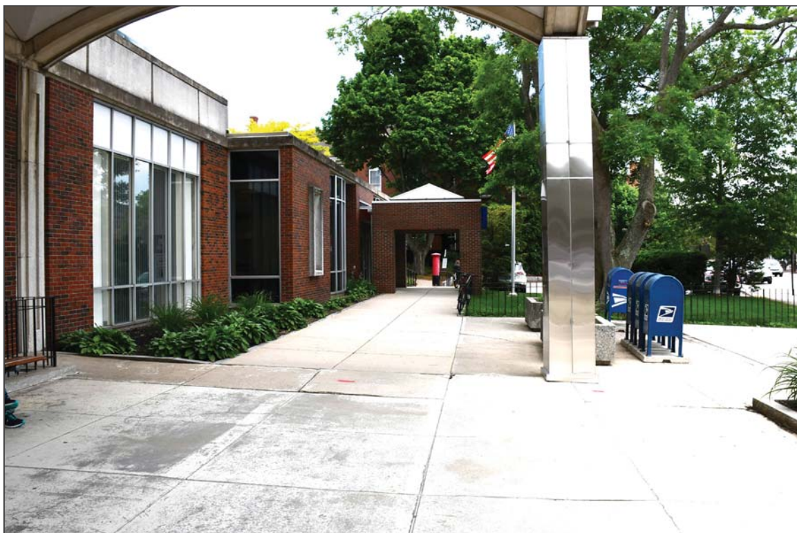
4. South elevation, facing east
