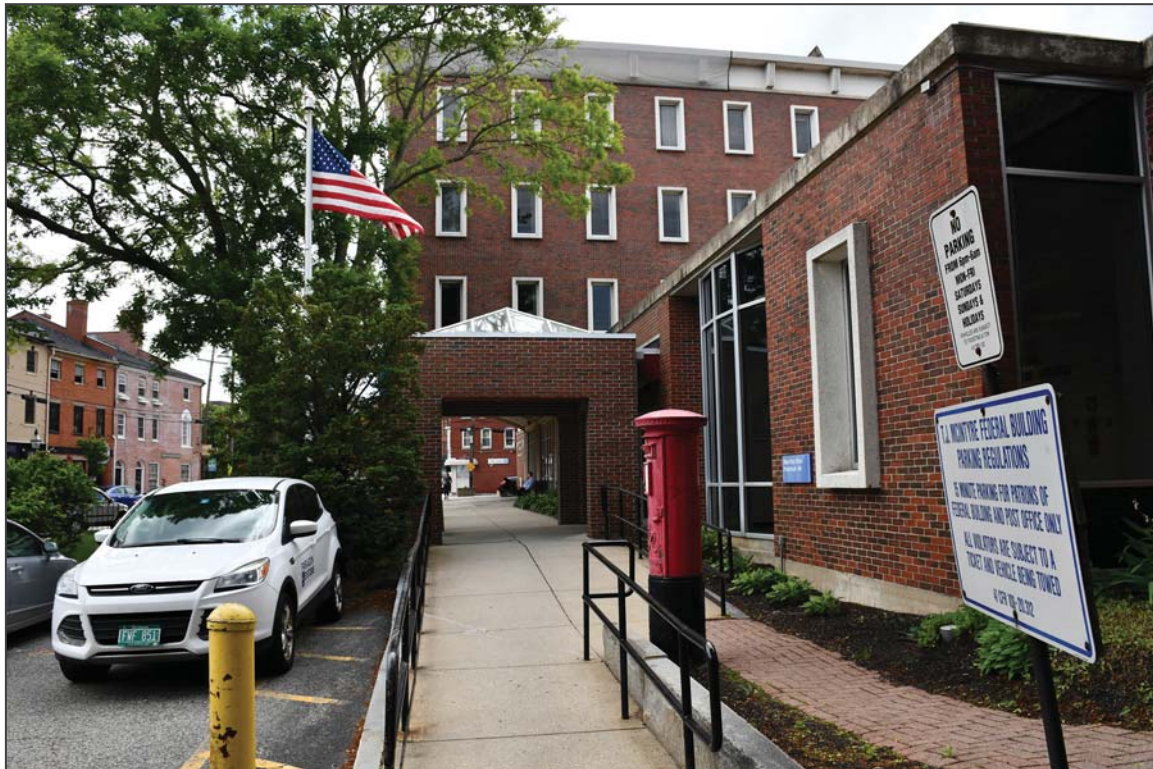
7. East and south elevations, facing west
