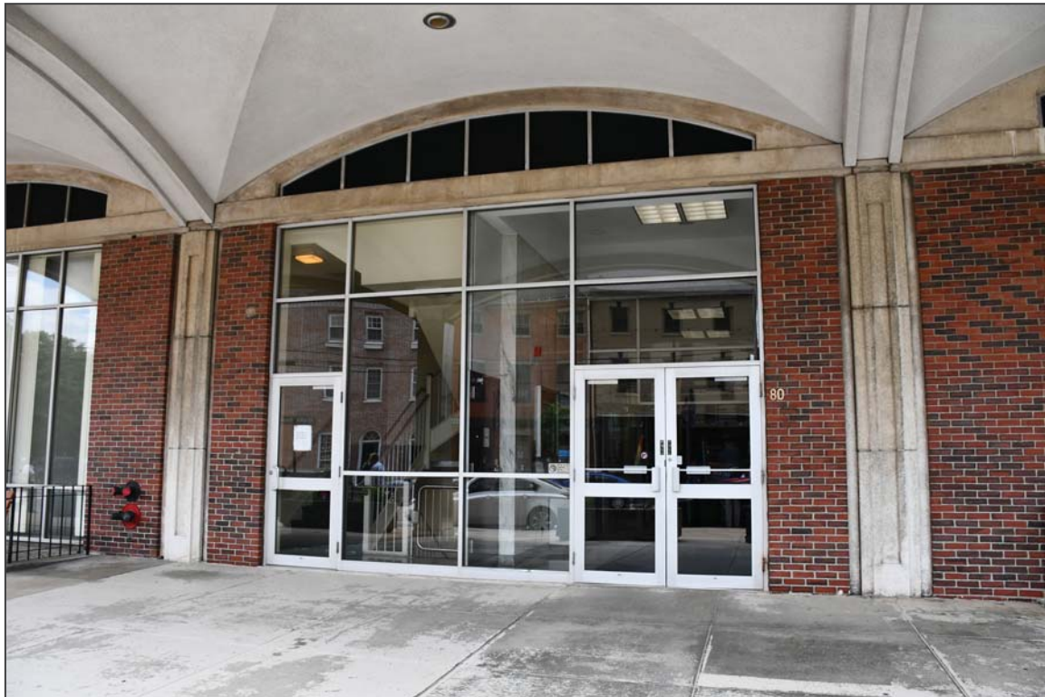
3. South elevation, facing north
