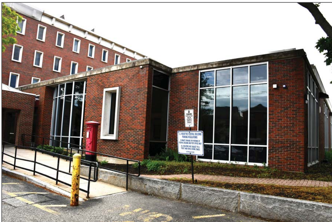
8. East and south elevations, facing northwest
