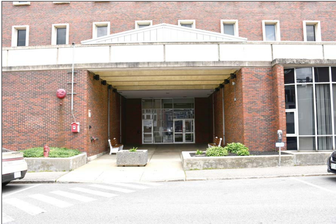
23. West elevation, facing east
