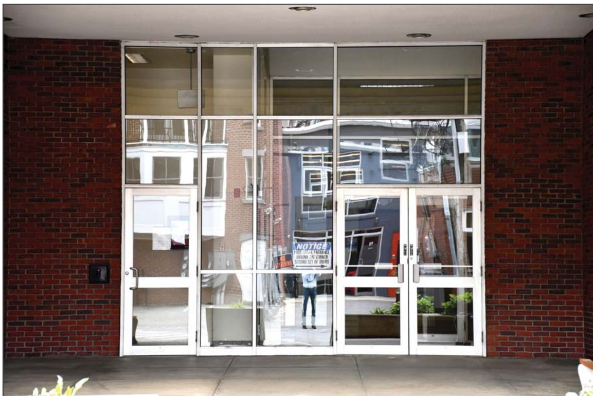
24. West elevation, facing east
