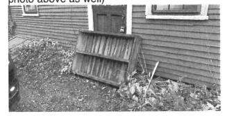
3) Remove existing wooden ramp leading in back of building (believe it was used by past owner to roll inventory (antiques) in an out of the building. It is old, weathered and in disrepair. We plan on landscaping it with cobbled stone and green space.
