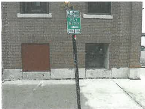
GAS METER AT NORTHWEST CORNER
