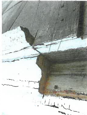
EXISTING WINDOW TRIM
