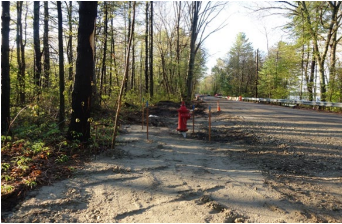
Picture 1: Addition of fire hydrant with waterline work.
