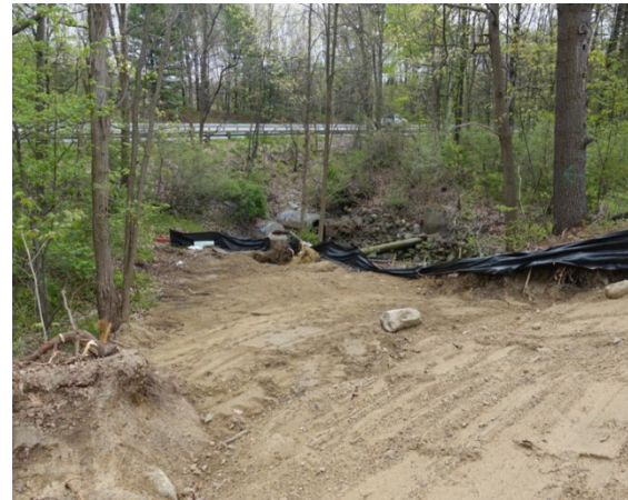
Picture 2: heavy equipment is needed to move heavy materials
