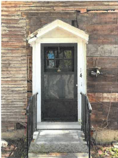
EXISTING FRONT ENTRY AFTER SIDING REMOVAL
