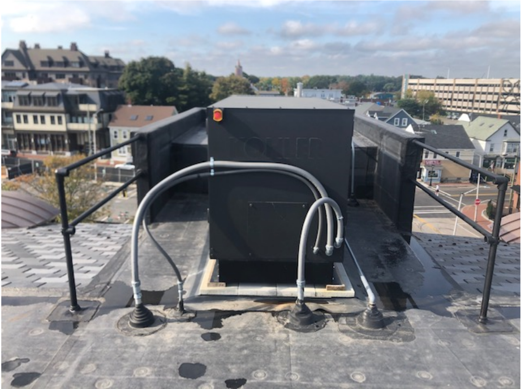
Rooftop generator with safety railing installed
