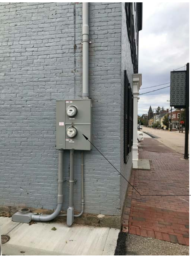
5. INSTALLATION OF (2) ELECTRICAL METERS
