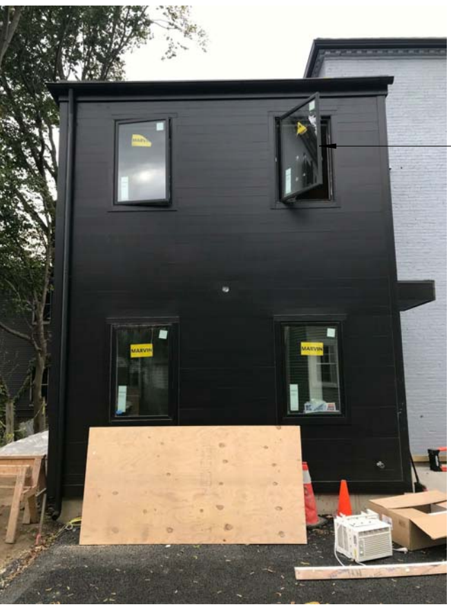
7. INSTALLATION OF (1) ADDITIONAL APPROVED MARVIN WINDOW
