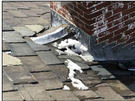
P4: EXISTING SHINGLE CRICKET TO BE REPLACED WITH A NEW FLAT SEAM COPPER CRICKET.
