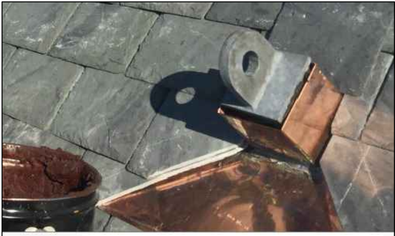
EXAMPLE OF FLAIED TRIMMED SLATE AT PENETRATIONS
