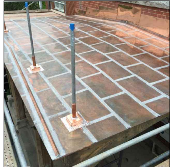
INSTALLED FLAT SEAM COPPER EXPECTATION
