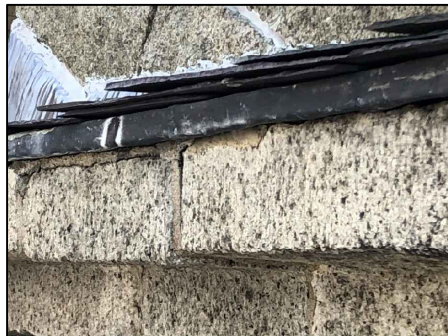
P2: EXISTING RAKE DETAIL SHOWING THE ENCAPSULATED WOOD DECK EDGE.
