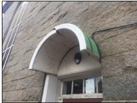
P6: EXISTING CANOPY TO BE RECREATED. PROVIDE NEW MATERIALS TO REBUILD.
