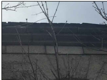
P7: EXISTING JOINTS IN THE TOP COURSE OF THE EXISTING FACADE TO BE RE-POINTED BY A MASON CARRIED BY THE ROOFING CONTRACTOR.
