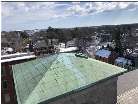
P1: FLAT SEAM STEEPLE ROOF WITH ROOF HATCH.
