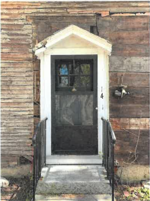
EXISTING FRONT ENTRY AFTER SIDING REMOVAL
