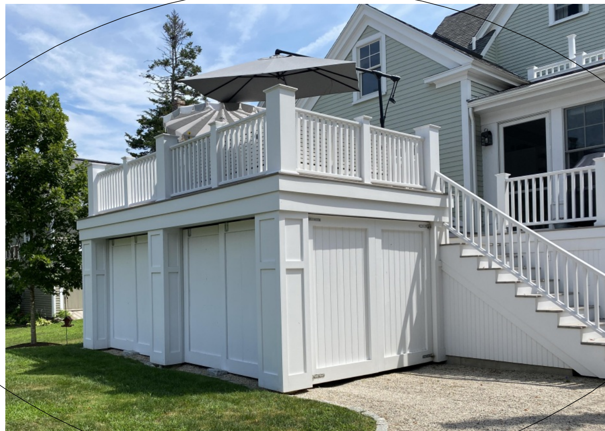
STORAGE AREA UNDER DECK REFERENCE FROM 11 SOUTH STREET NOTE: MATCHING PANELS ONLY - FLUSH INSTALLATION
