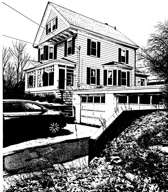
EXISTING CONDITIONS (VIEW FROM RIGHT)
