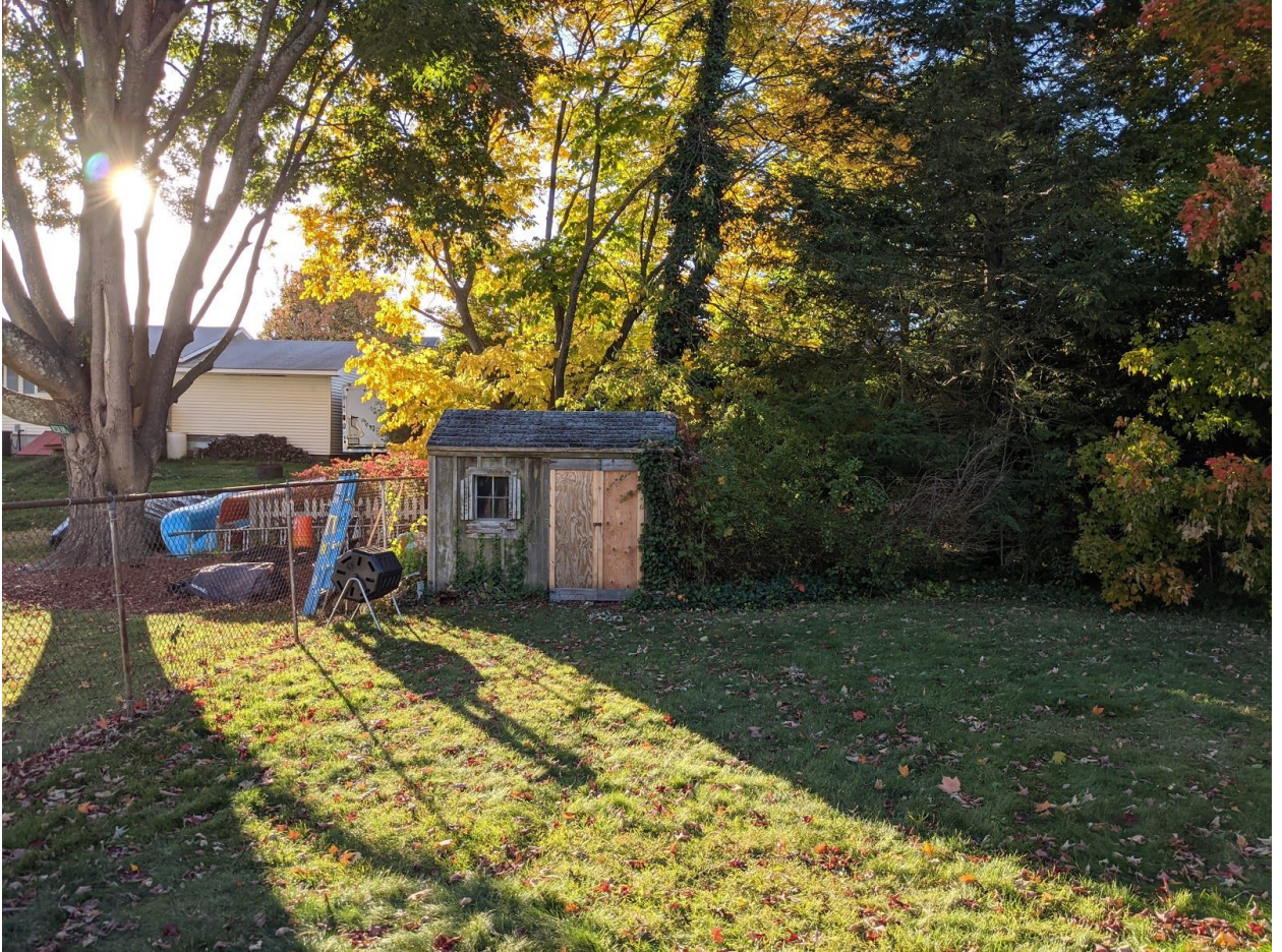
Shed in back left corner of lot
