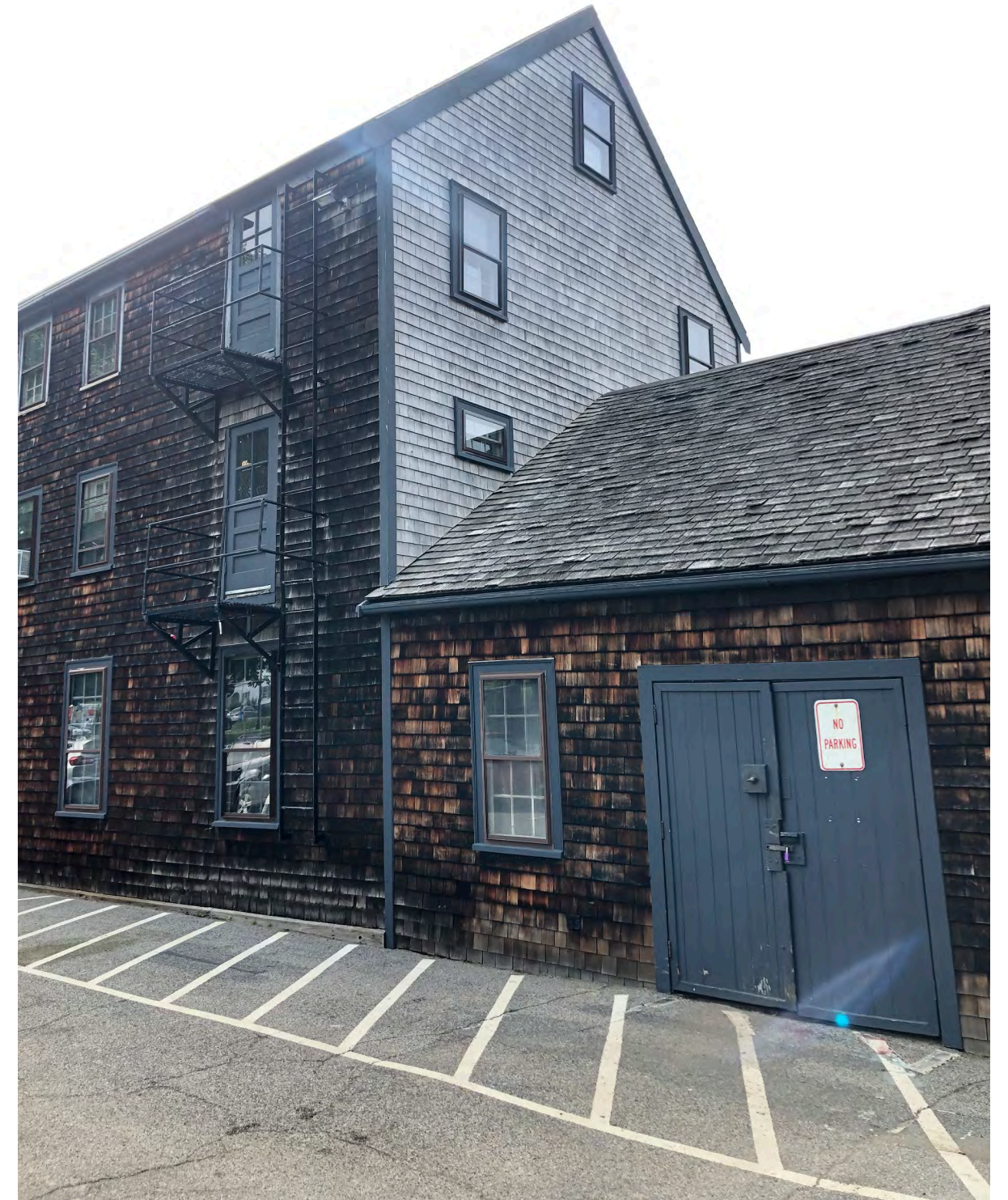
South Elevation - Emergency egress stair and connection to Lean-To addition
