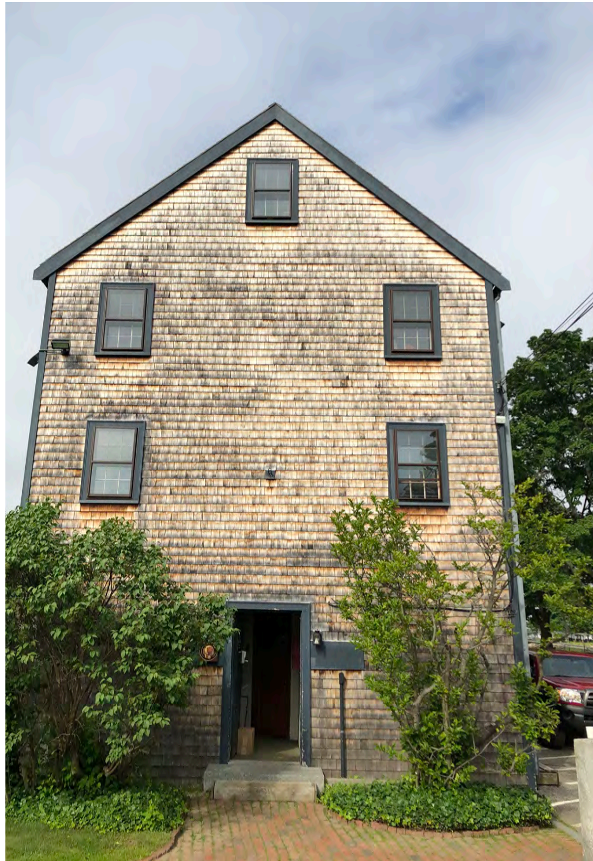
West Elevation - Entrance to building
