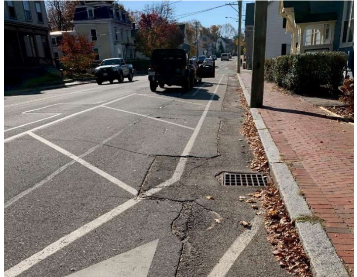
Figure 1: Photo of pavement seam and catch basin at start of southbound bike lane, and parked car with open door visible
