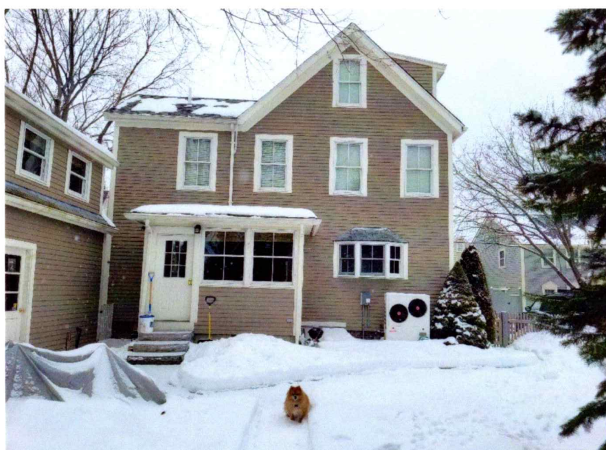
VIEW OF REAR ELEVATION AT NEW BAY
