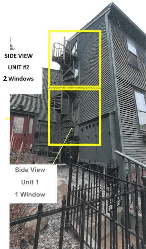
93 HIGH STREET SIDE VIEW OFF HIGH
