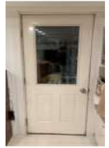
Previously-approved 2x4-frame existing metal door
