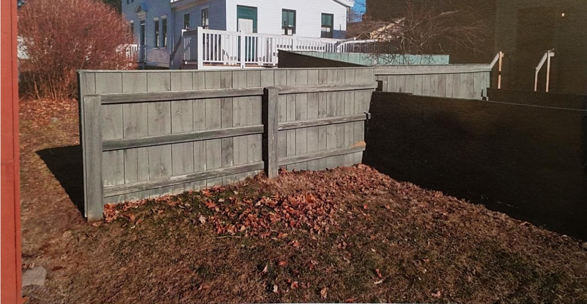
Example of Solid board fence Lear West fence (S. Banke location)
