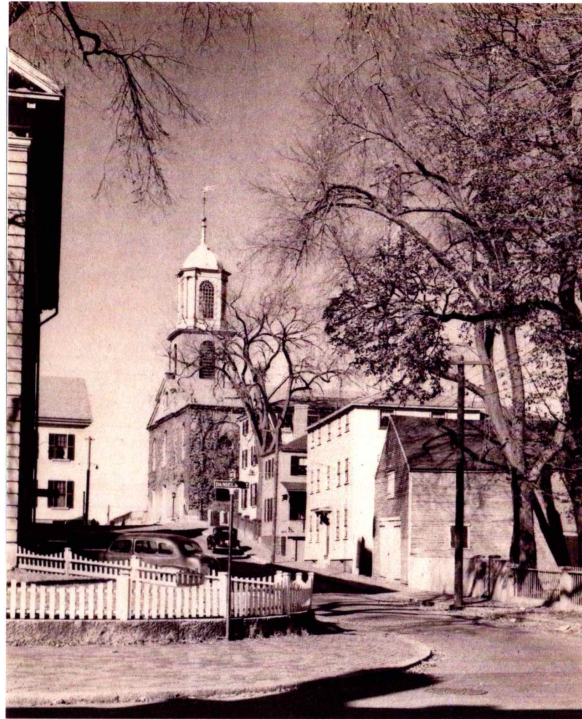
PHOTO OF ORIGINAL CARRIAGE HOUSE
