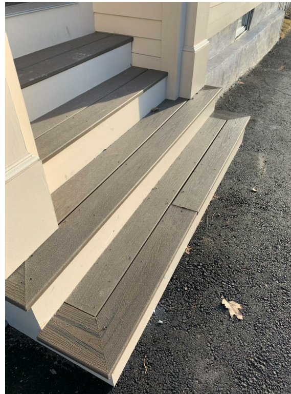
IMAGE OF REPAIRED STAIRS
