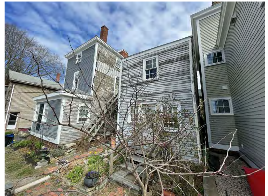
VIEW OF EXISTING SOUTHEAST ADDITION
