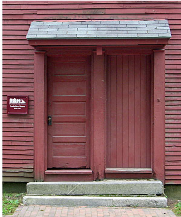
1 SOUTH WEST FRONT DOORS
