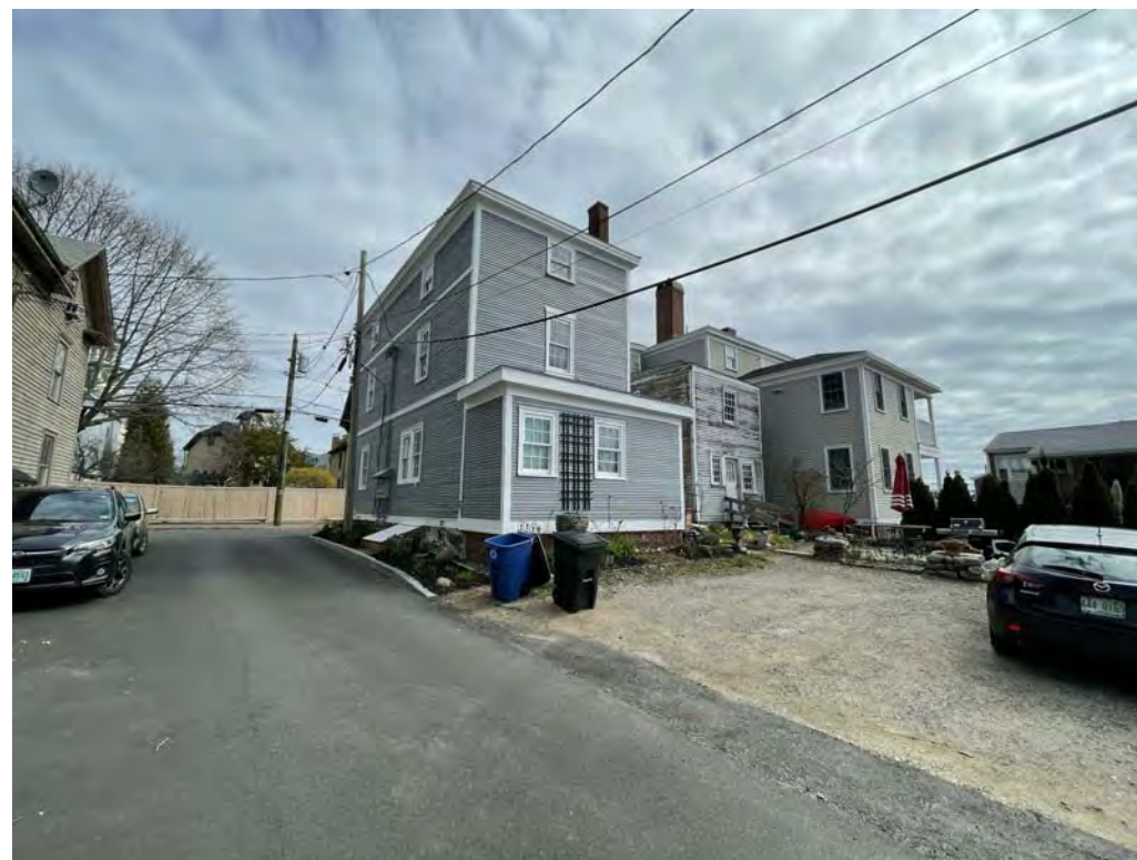
REAR OF BUILDING FROM FRANKLIN STREET
