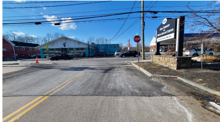
Albany Street looking west at the intersection
