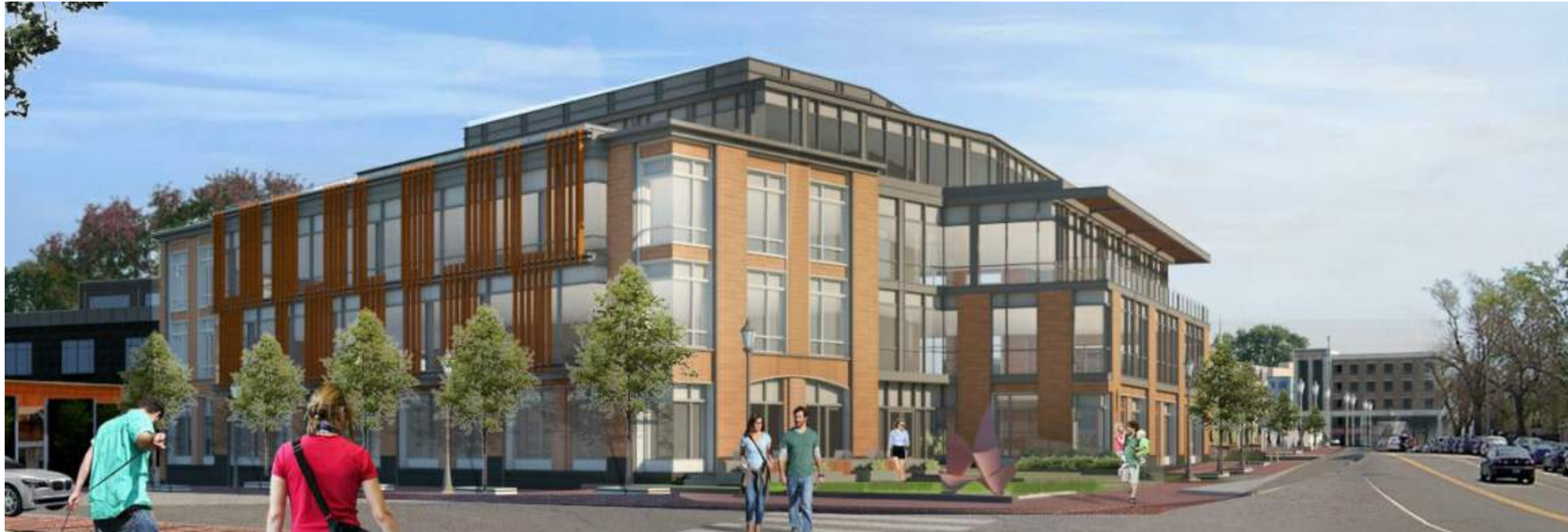
OFFICE BUILDING CURRENTLY UNDER CONSTRUCTION - 145 MAPLEWOOD AVENUE
