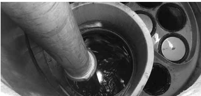
Vacuuming Sump Through MAW
