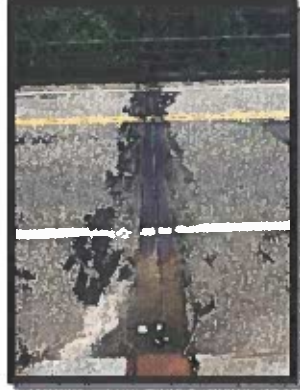
East Expansion Joint
