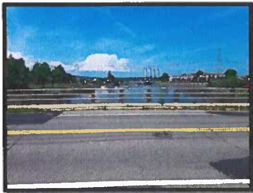
Typical Pavement Condition
