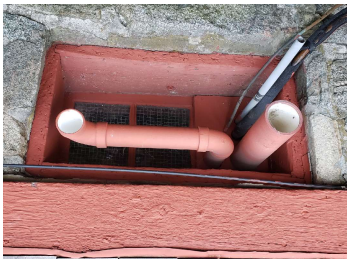
Existing furnace Intake/Vent
