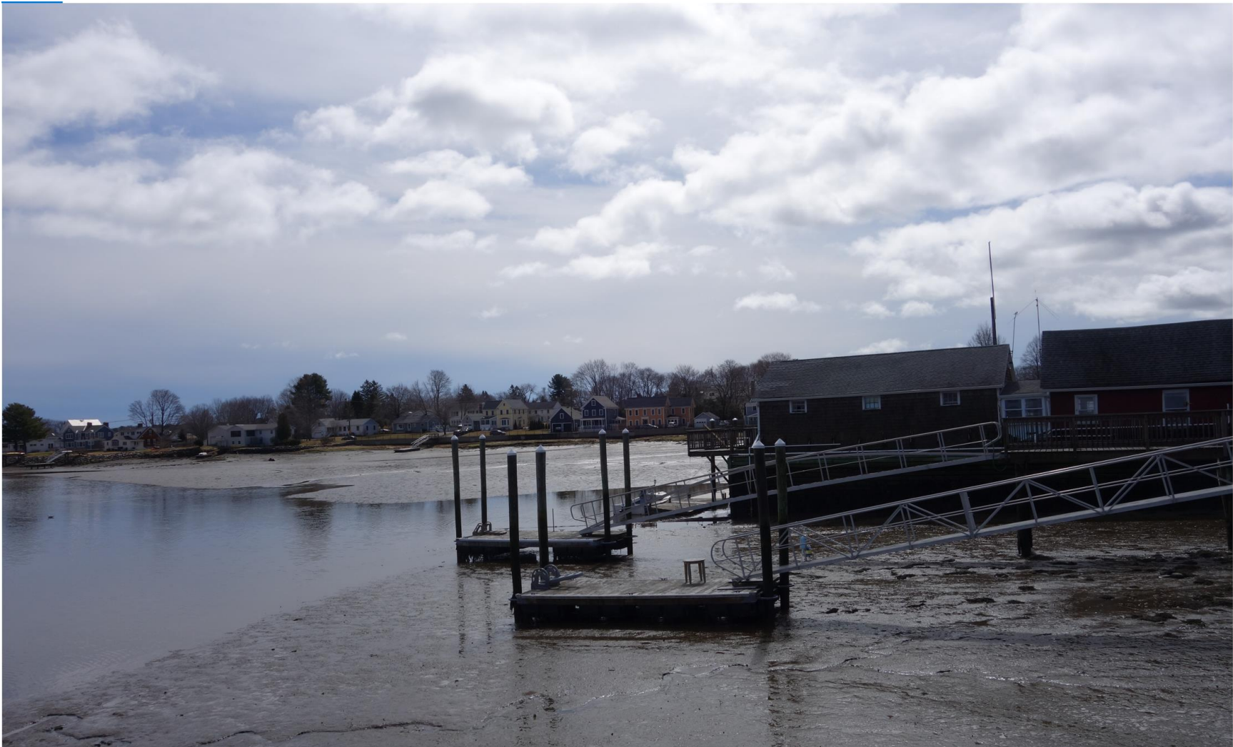
Photographs Demonstrating the View of Homes and Buildings from the Shoreline – 57 Salter Street, Portsmouth
