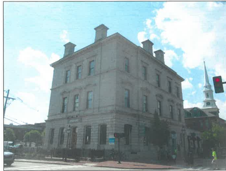
EXISTING SOUTH EAST BUILDING CORNER
