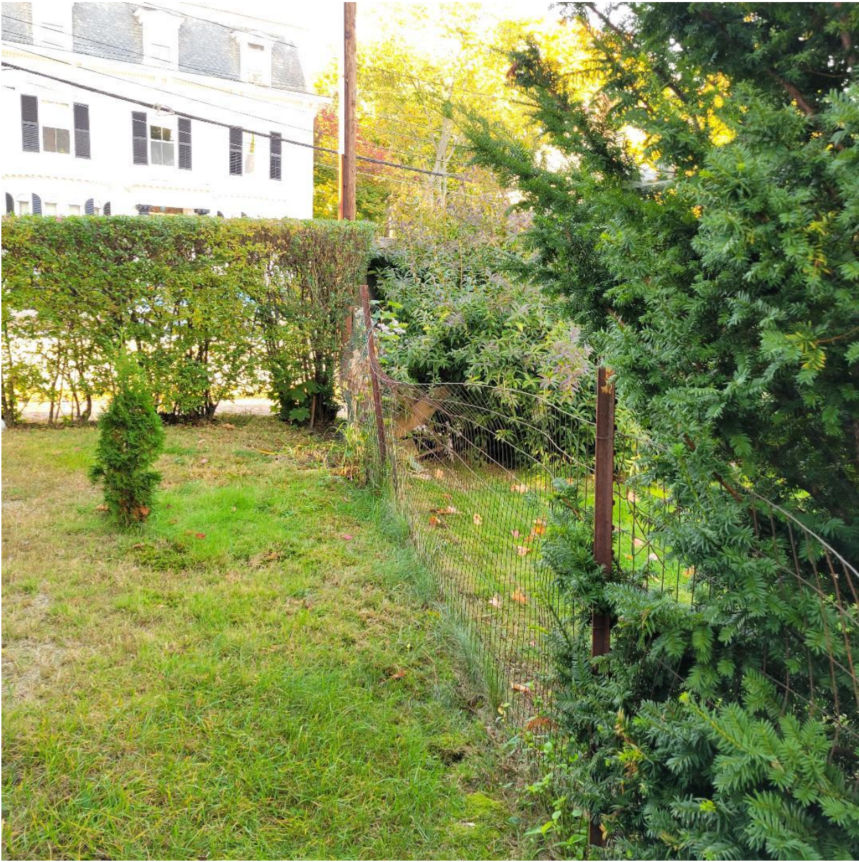
Existing fence to be replaced
