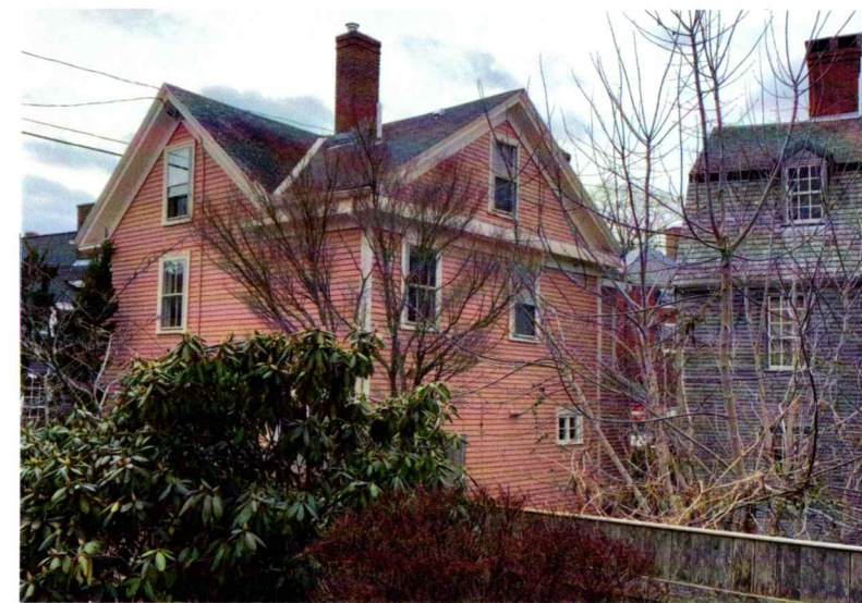
VIEW FROM MANCOCK STREET
