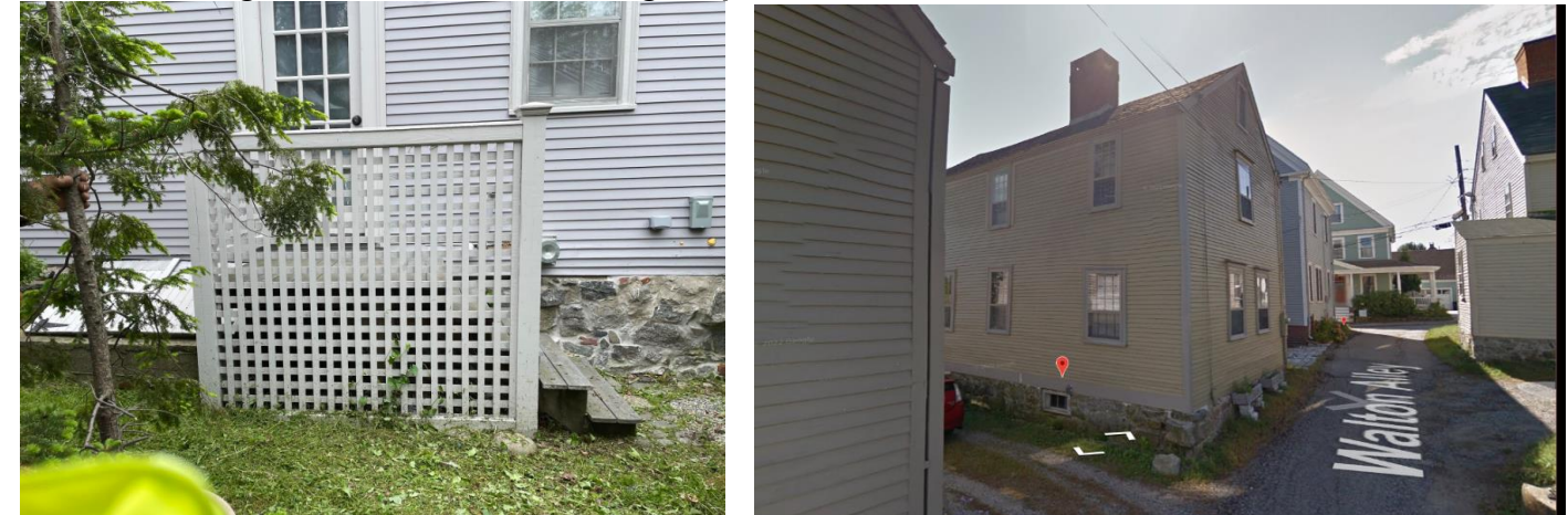
Rear Elevation and Streetscape View
