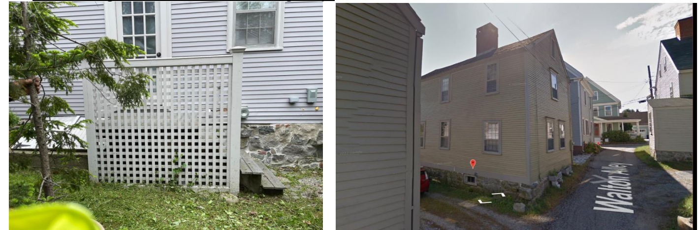
Rear Elevation and Streetscape View
