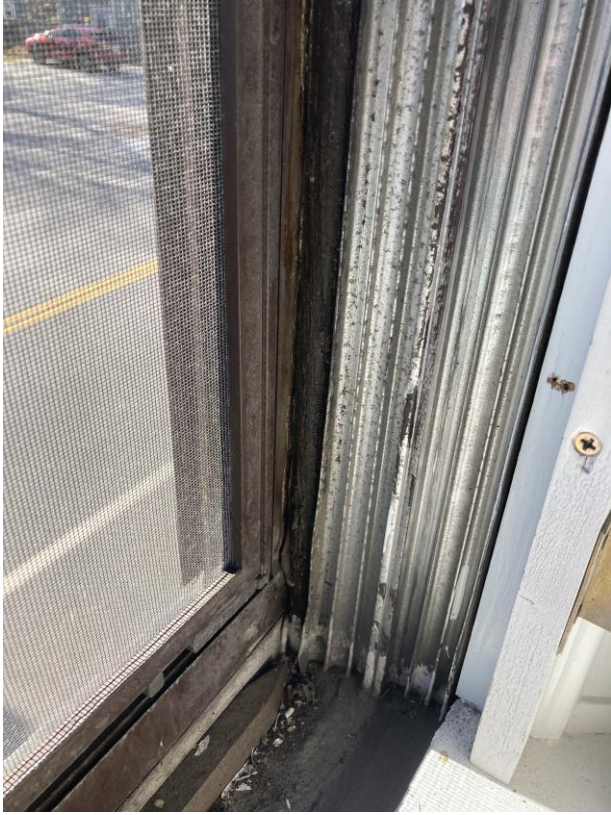
Existing window conditions
