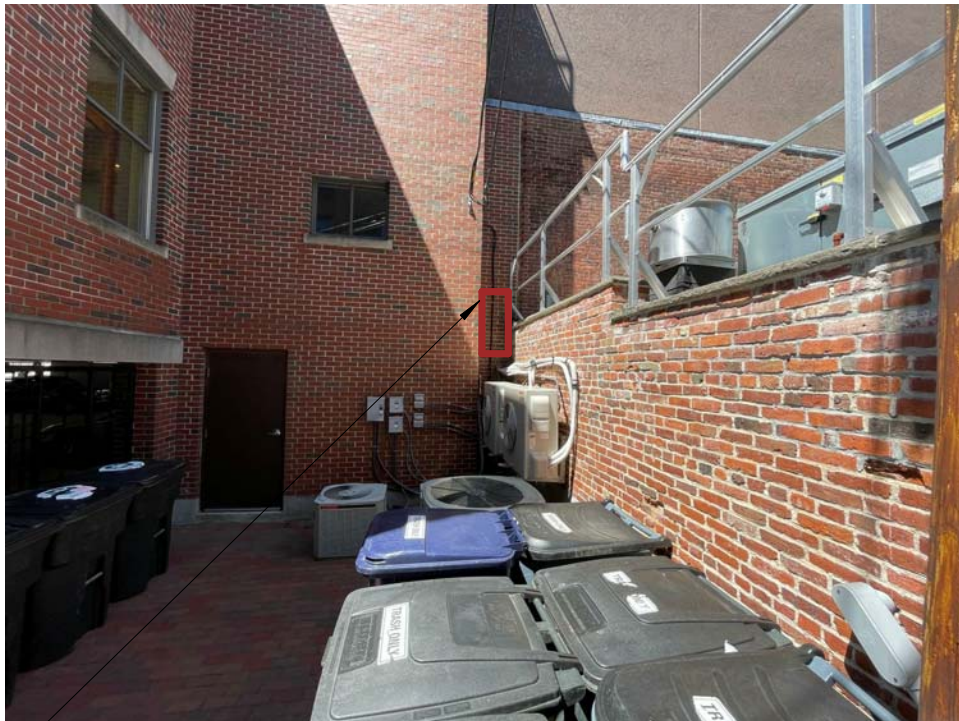
LOCATION OF 18" x 30" INTAKE LOUVER, PAINTED TO MATCH ADJACENT BRICK, REFER TO SKH-1 AND APPENDIX
