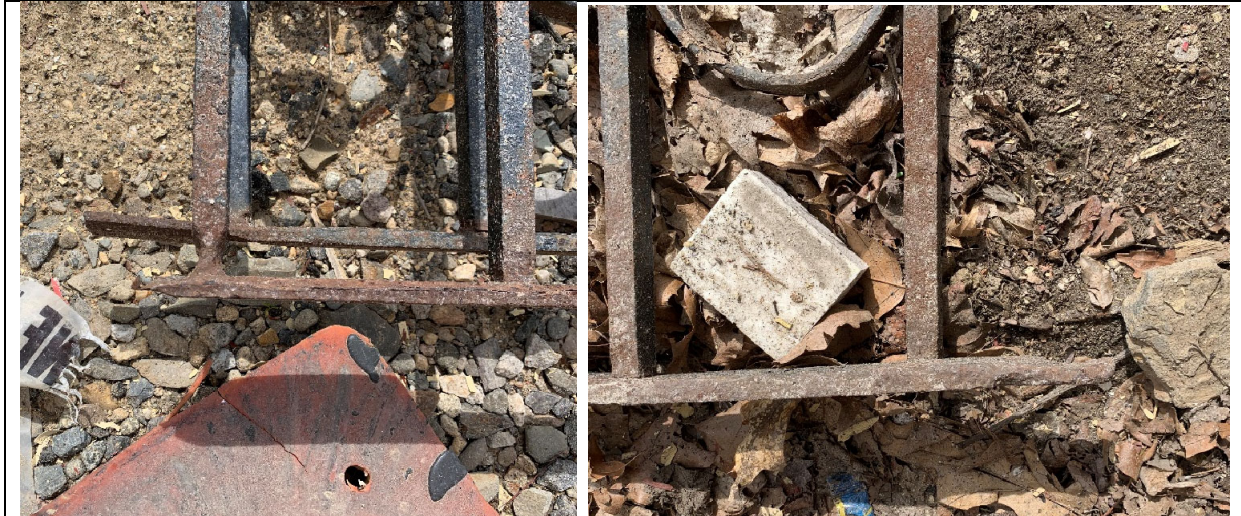
Current Fence – Rust / metal missing at connection points
