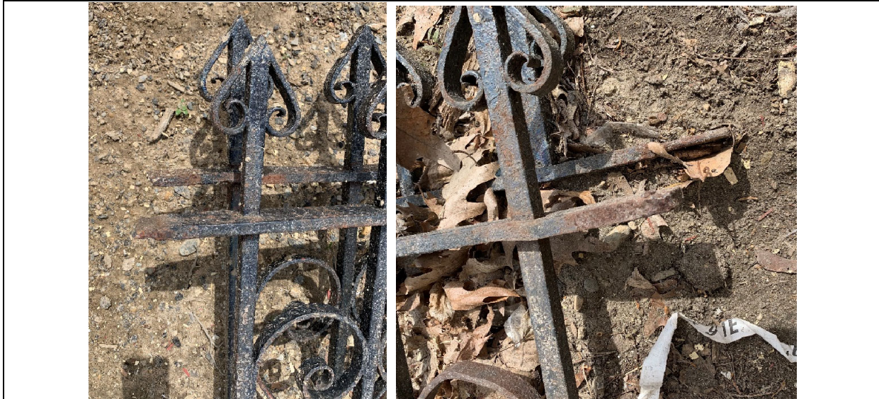
Current Fence – Rust / metal missing at connection points
