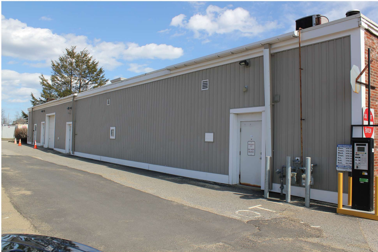
ELEVATION FACING RAILROAD TRACKS
