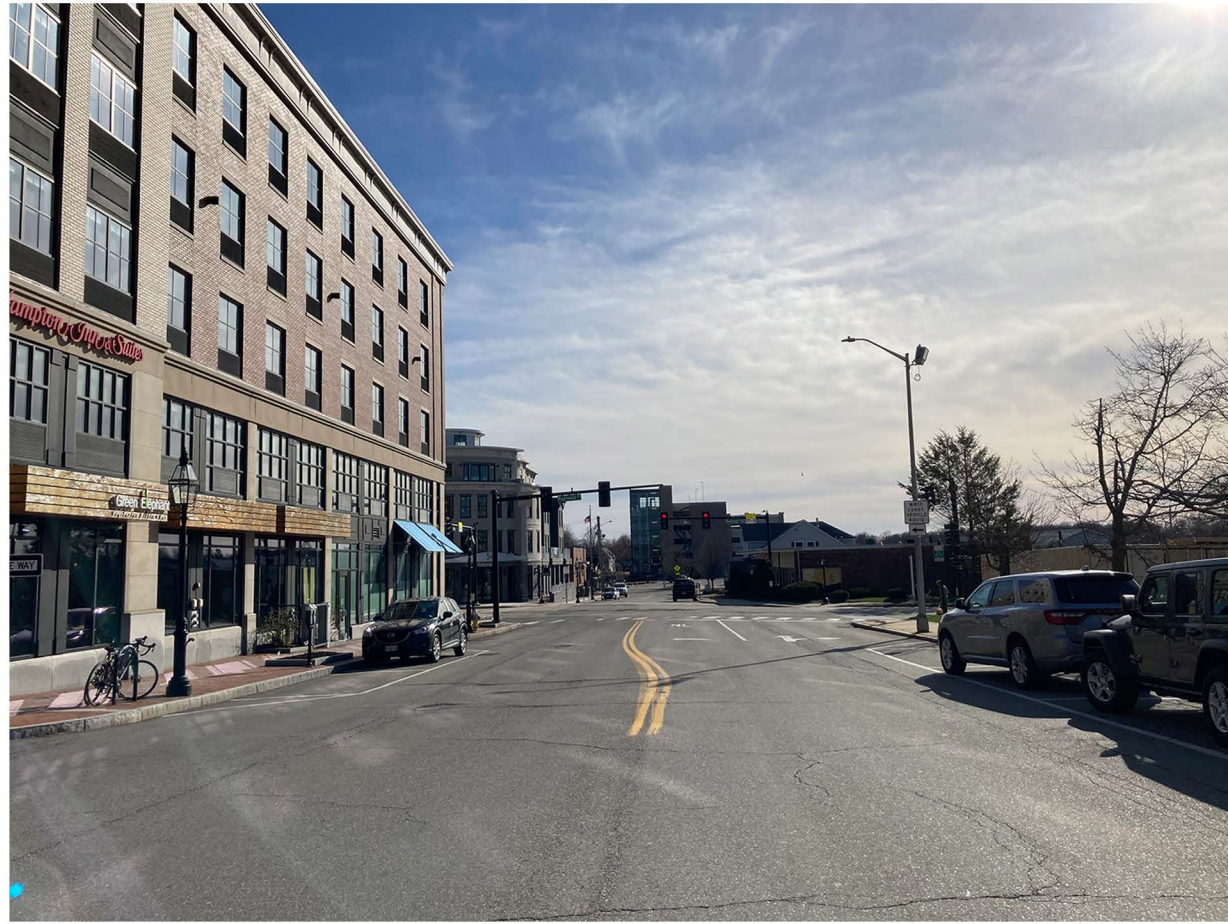
E. VIEW FROM DEER STREET TO FOUNDRY GARAGE
